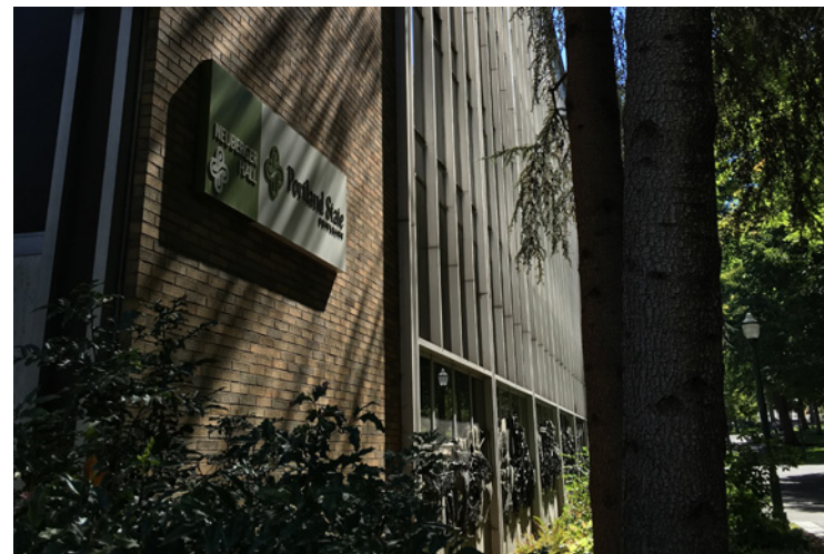
NEUBERGER HALL NORTHWEST FACADE DETAIL
