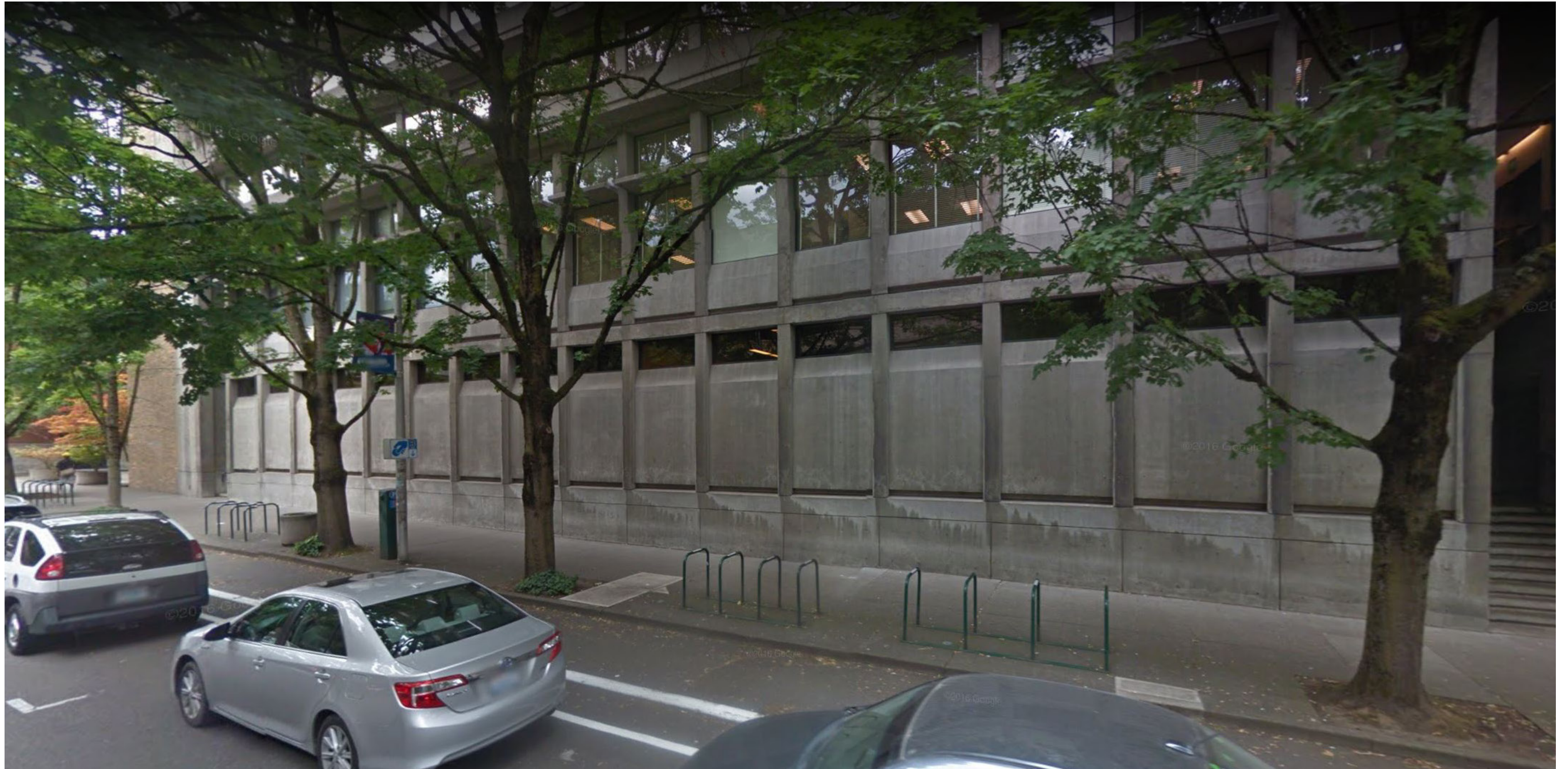
EXISTING EAST FACADE
