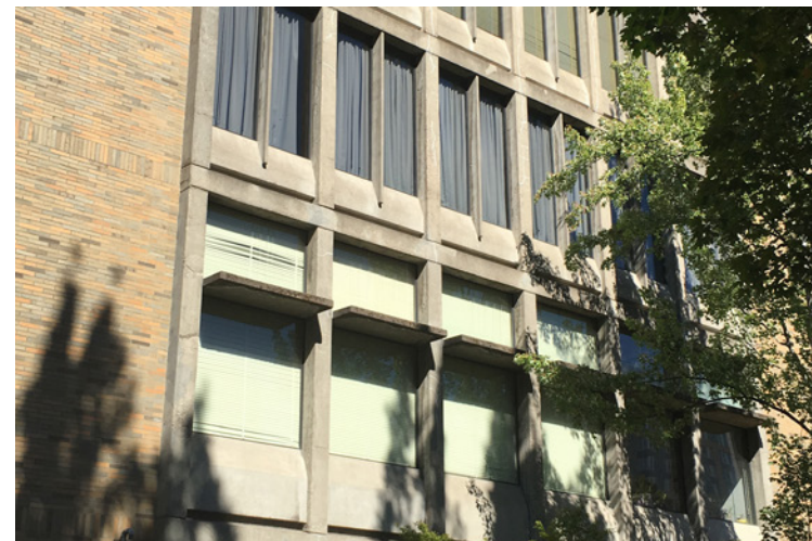
NEUBERGER HALL EAST FACADE GROUND FLOOR
