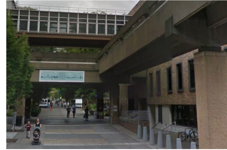
SW HARRISON ST PEDESTRIAN BRIDGES FACING WEST
