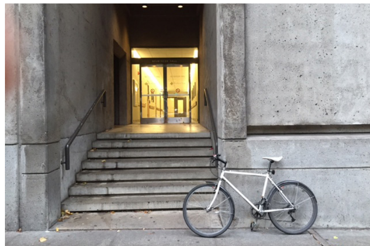
SW BROADWAY EXIT CORRIDOR
