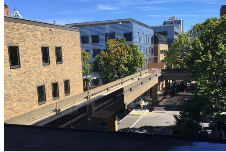
SW BROADWAY PEDESTRIAN BRIDGE FACING EAST
