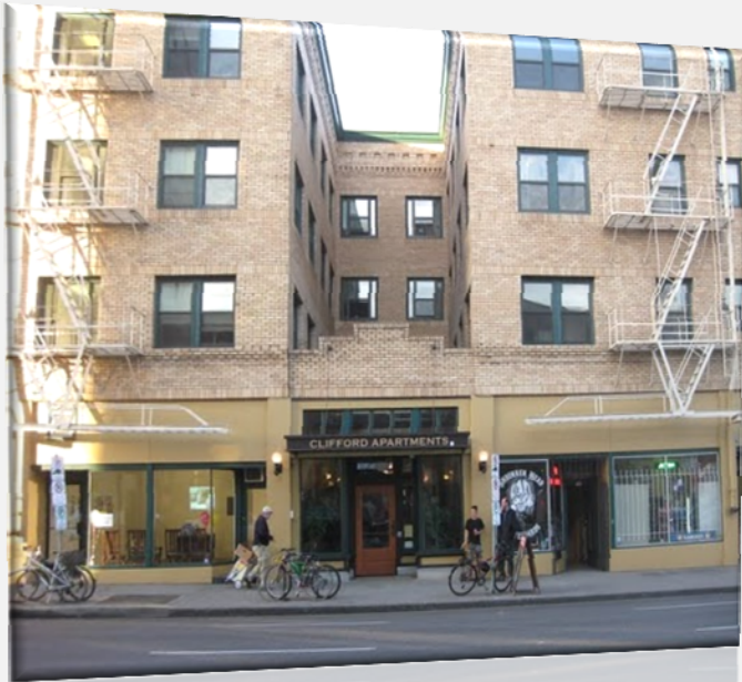
The Clifford provides 88 units of affordable rental housing . Address: 527 SE Morrison Street
