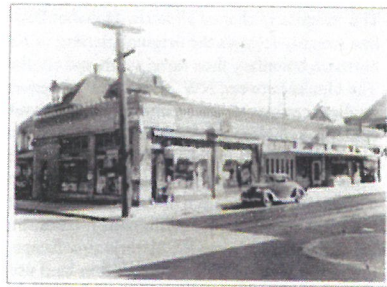
Looking southeast at 622 NW 23rd Avenue
