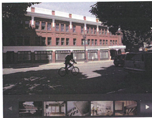
The facade facing NW 2nd Avenue just north of Burnside. Innovative Housing has remodeled two Old Town buildings into 62 studio and one-bedroom apartments. 52 of which are affordable housing. Salvaged material and original features from the Erickson Salove and Erb Hotel Buildings, built in 1912, were retained for use throughout the new
