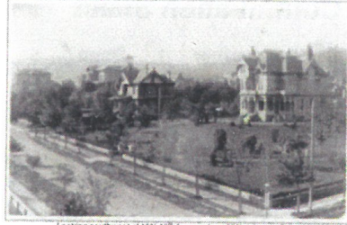
Looking southwest at NW 10 th Avenue from NW Johnson Street
