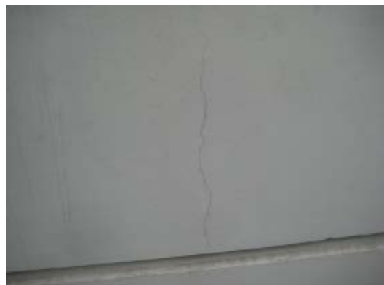
80. Concrete Cracking
