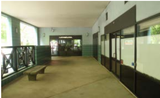
30. Recessed Storefront Assemblies at Loggia Level
