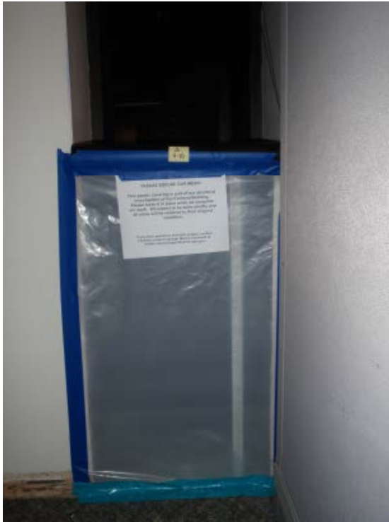
98. 9.10 (9 th floor, north elevation)
