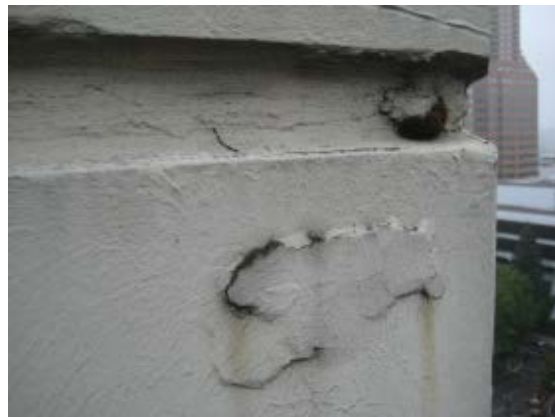
83. Concrete Spalling
