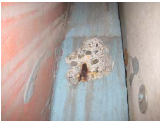
81. Concrete Spalling
