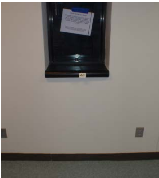
7. Test Site 4-10 Observation complete and wall repaired.
