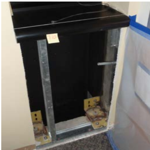
21. Interior Wall at Spandrel Panel
