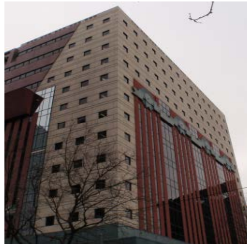
78. Concrete with Elastomeric Coating (beige and red)
