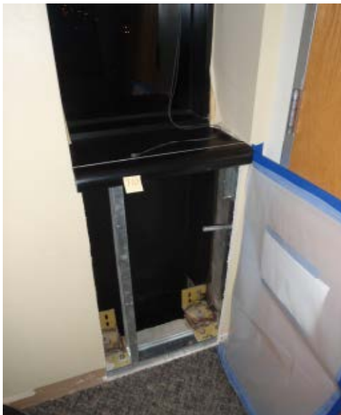
95. Test Location 7.10 (7 th floor, south elevation)
