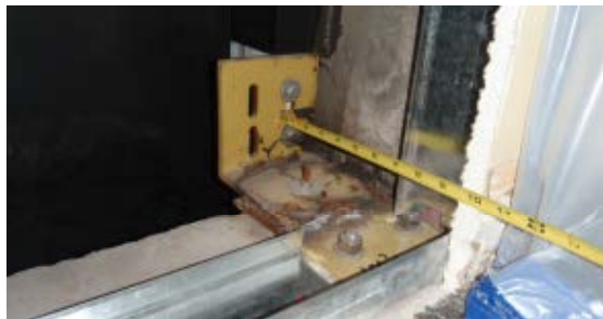
14. Curtainwall Connection Detail
