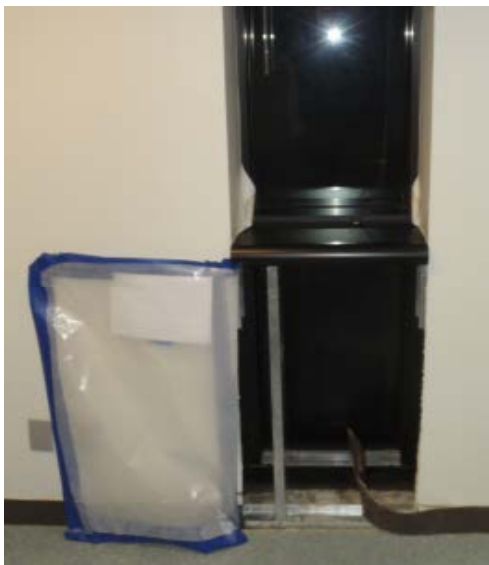
91. Test Location 4.10 (4 th floor, south)
