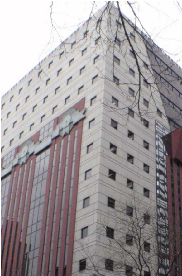
23. Punched Windows in Concrete Wall
