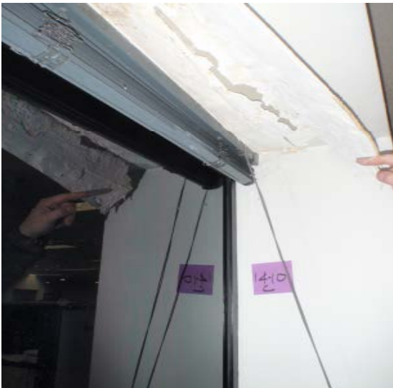
107. 14.10 Window at Adjacent Window
