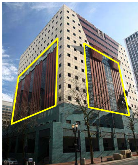
15. Curtainwall Assemblies Identified
