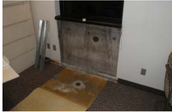
8. Test Site 11-1, 11-2 Interior finishes removed and concrete core samples taken.
