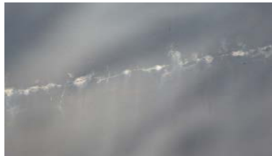
79. Concrete Cracking
