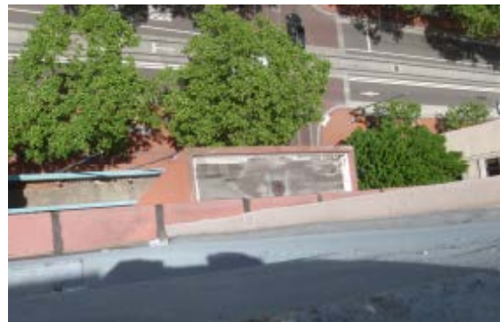
20. Roof at Column Capital
