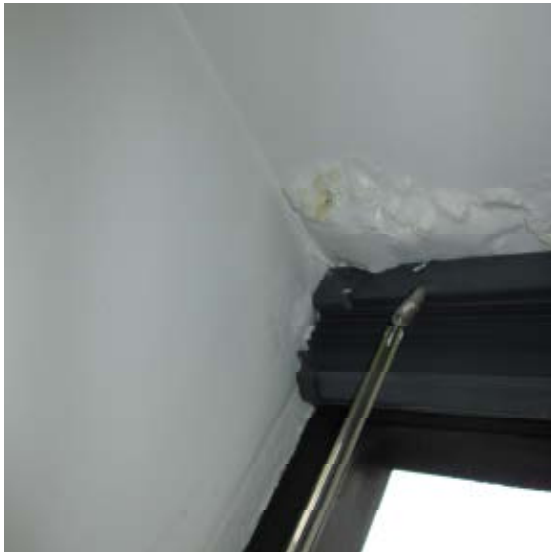
90. 14 TH FLOOR WEST WINDOW HEAD
