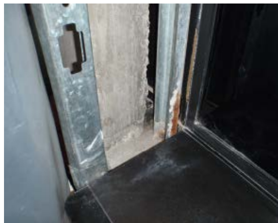
105. 14.10 Window Sill at South End
