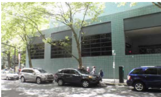
31. Surface Storefront Assemblies at Loggia Level
