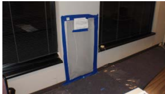
9. Test Site 15-4 wall opened for observation
