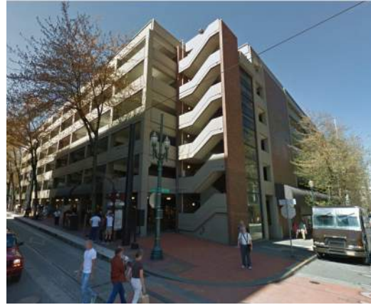
existing southeast corner
