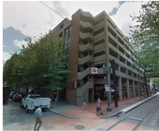
existing northeast corner
