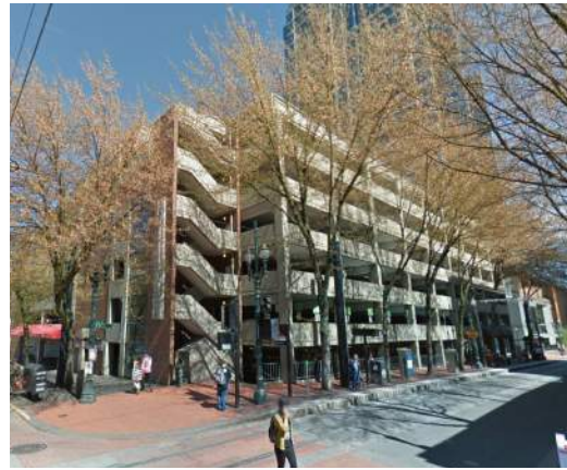
existing southwest corner
