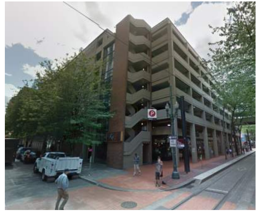
existing northeast corner
