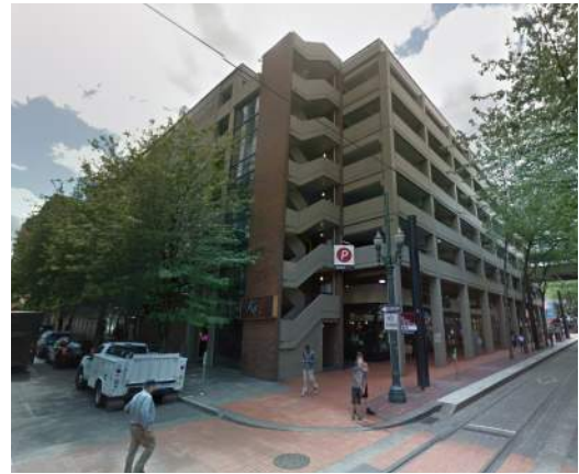
existing northeast corner
