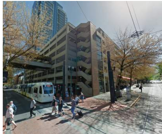
existing northwest corner
