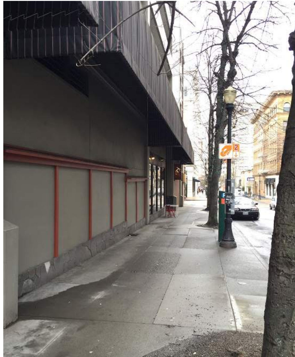
Existing facade along SW Ninth Avenue.
