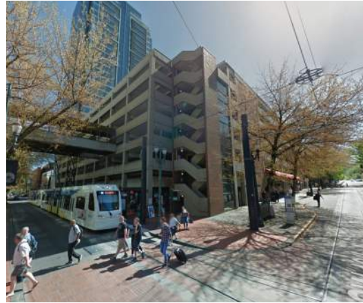
existing northwest corner
