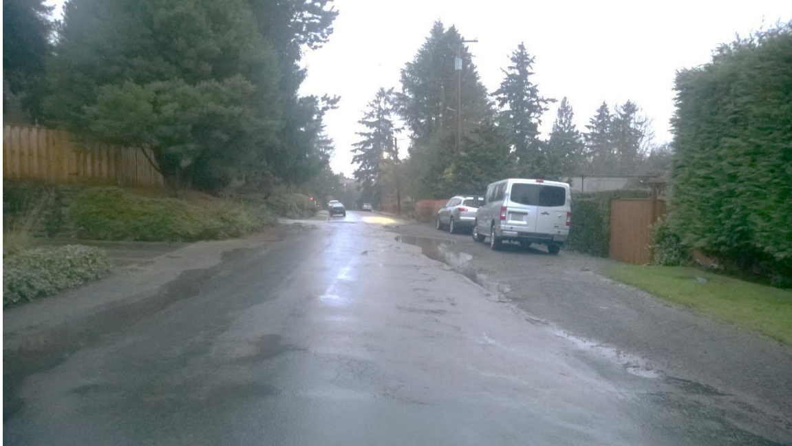
SW Hume Street, facing west at SW 11 th Avenue. Under-improved - lacking sidewalks, curbs and gutters.
