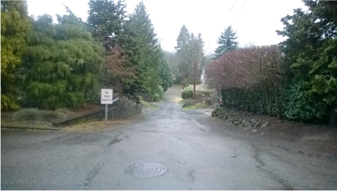
SW 12 th , facing north at SW Hume Street. Under-improved, narrow, and lacking curbs, gutters and sidewalks.
