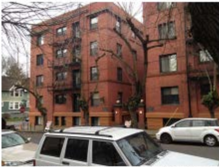
Across 15 th St. (west). Apartment complex. Zoned CM
