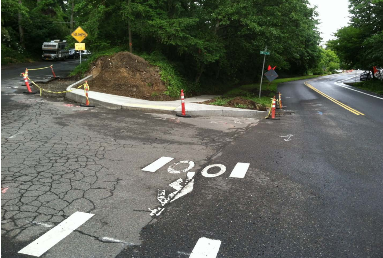
SW 7 th and Terwilliger Intersection Looking North (note sidewalk in the path of future bike lane alignment)
