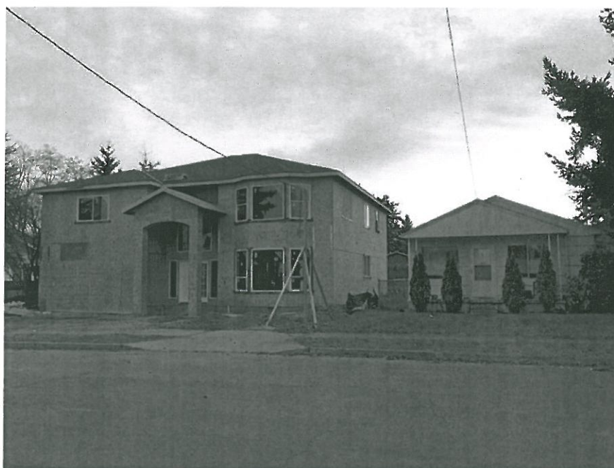
New homes are being built in established neighborhoods throughout Portland, particularly in the Southeast. Photographed here, a new home nearly four times the size of houses around it is being constructed in Mt. Scott-Arleta. (Melissa Binder/The Oregonian)
