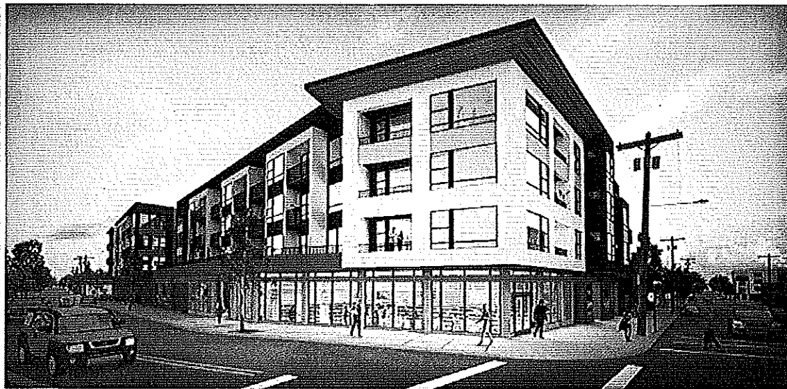
127-unit building with Green Zebra grocery planned for SW corner of 50 th and Division
