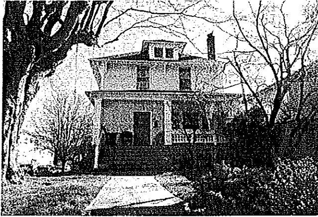
704 SE 29 th Year built: 1910 Description: single-family residential Current zoning: R5 Proposed zoning R1
