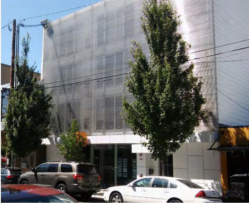
View of building from SE Division St
