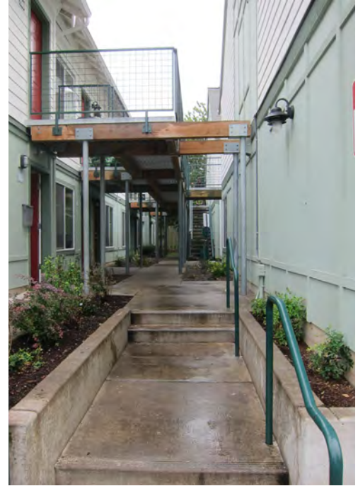
Internal walk between apartment buildings
