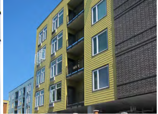
Cladding on western facade of building
