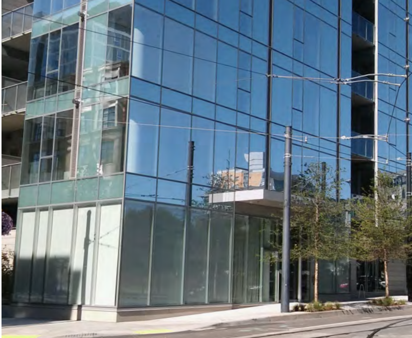
Ground floor at southwest corner of building as of August 2016
