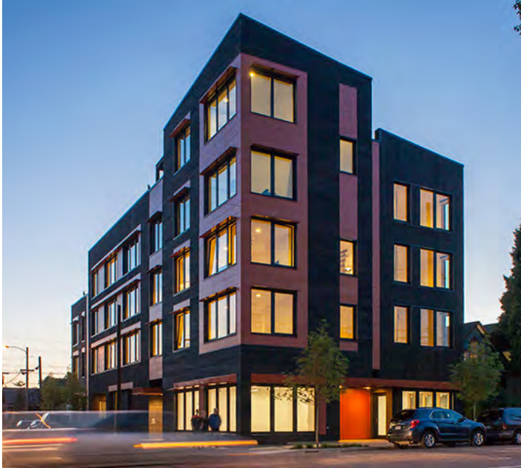
View of southeast corner of building
