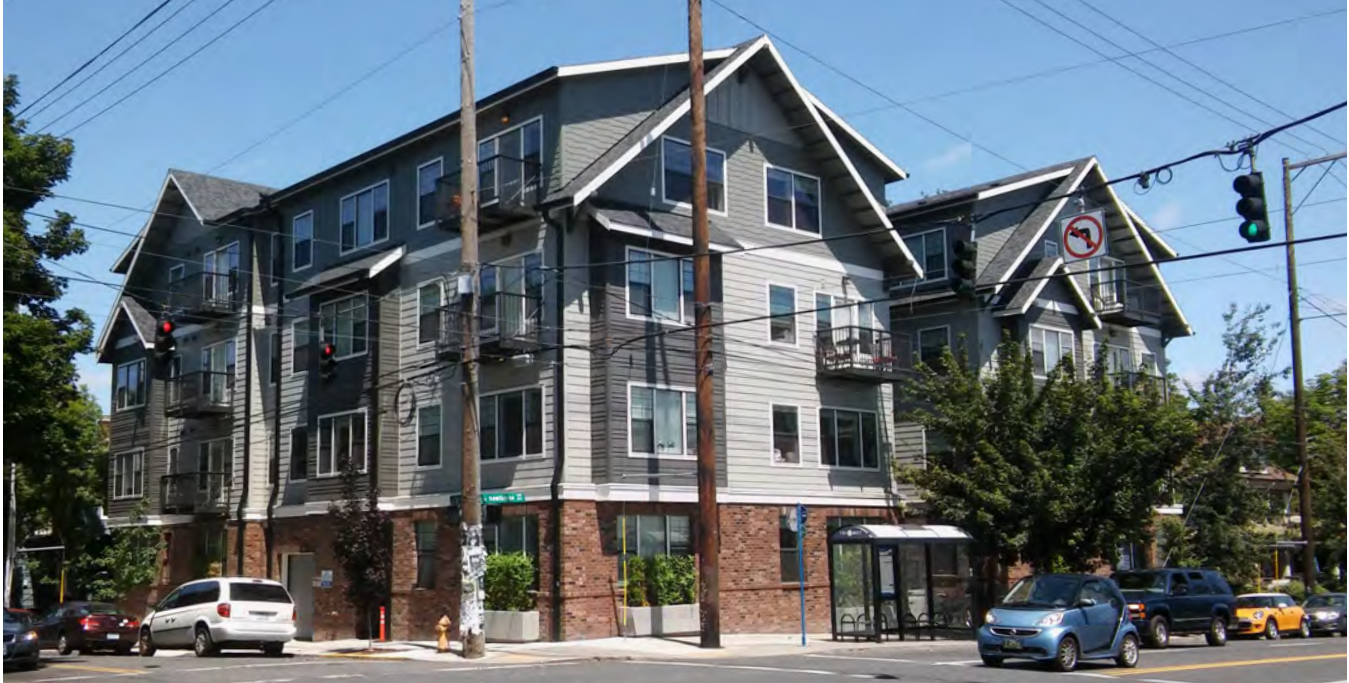
View of building from SE Hawthorne Blvd
