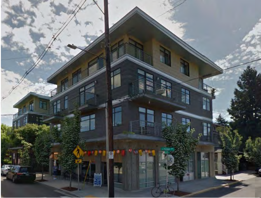
View of building from SE Division St
