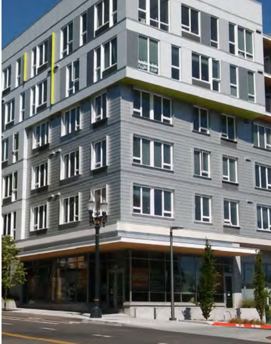
View of western corner
