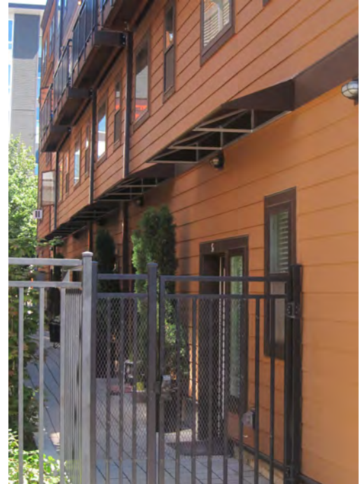
View of alleyway access to ground floor units
