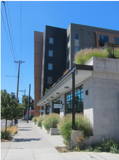
The design of the first 30 feet of a building are particularly important to the pedestrian experience; a 12 foot first floor height for residential and a 15 foot height for mixed use buildings is recommended
