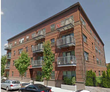
This building promotes permanence by using high-quality materials and attention to detail. Inset window glazing and the use of window sills create a sense of authenticity.
