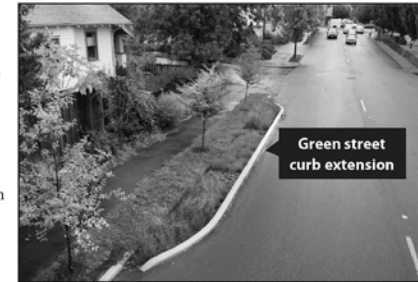
A green street planter is a small rain garden that collects stormwater runoff from streets.
