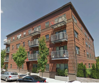
This building promotes permanence by using high-quality materials and attention to detail. Inset window glazing and the use of window sills create a sense of authenticity.
