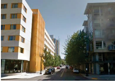
An industrial aesthetic was common throughout the examples, but at times the design looks out of place if not inspired by industrial buildings in the neighborhood.
