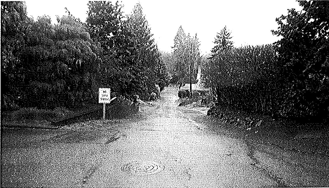
SW 12 th , facing north at SW Hume Street. Under-improved, narrow, and lacking curbs, gutters and sidewalks.
