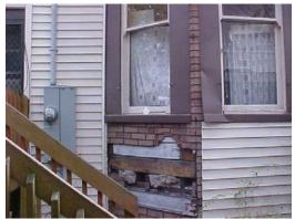
Inspector's photo of broken window and missing siding
