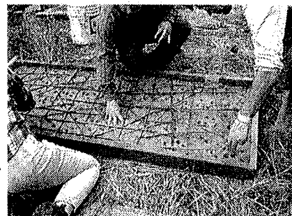
Placing reinforcing willow branches in the cast of a thin panel.
