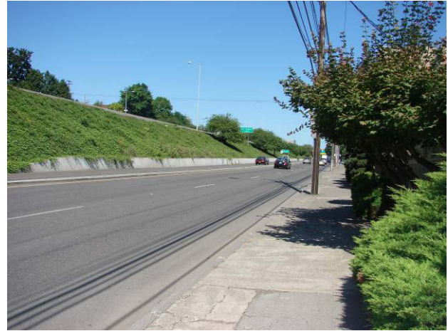
SW Macadam Avenue from near SW Abernathy Street, looking northbound.
