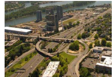
View of the west end of the Ross Island Bridge looking southbound.
