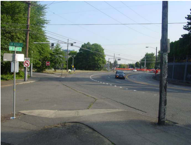
The existing ramp from Macadam Avenue to Kelly Avenue comes in on the left in this photo. That ramp would be reconstructed and brought in further south to the Kelly/Porter intersection
