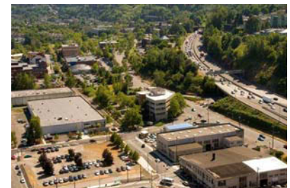
Views of North Portal area (top) and South Portal area (bottom)
