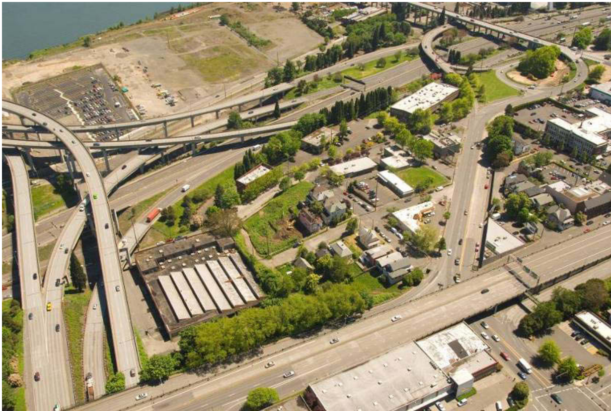
Aerial photo of the SW Kelly Avenue area where several of the motor vehicle projects focus to improve the North Portal access to the study area
