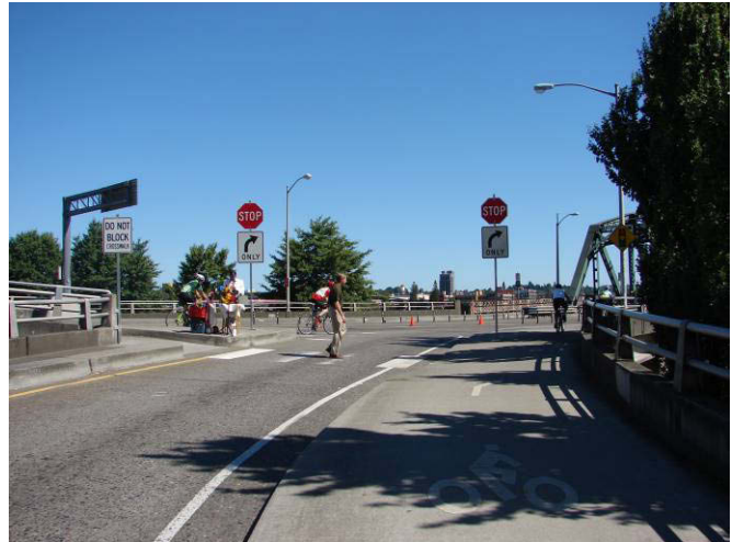
A view from the northbound SW Naito Parkway ramp onto the Hawthorne Bridge. This ramp would be widened to two lanes and a traffic signal placed at the intersection with the eastbound Hawthorne Bridge traffic.
