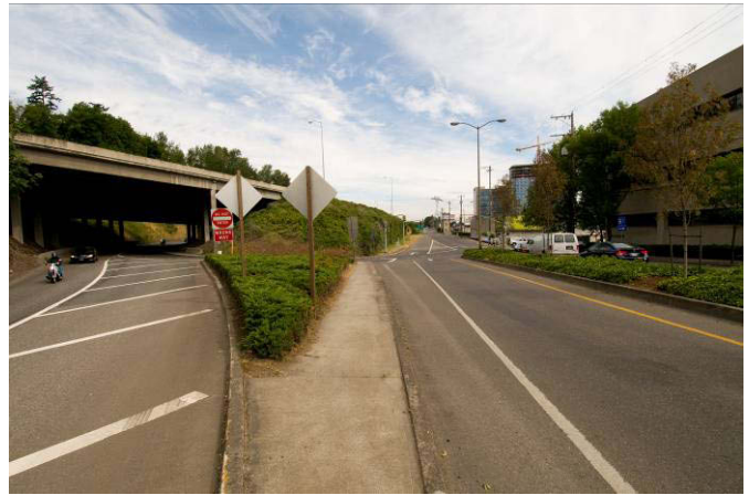
This photo is a northbound view on Macadam Avenue and shows the limited sight distance of southbound traffic on SW Hood Avenue approaching the SW Bancroft Avenue intersection.
