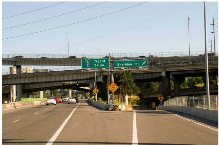
Looking southbound on SW Harbor Drive as the Southbound Harbor Drive ramp leaves the main roadway to SW Sheridan Street.
