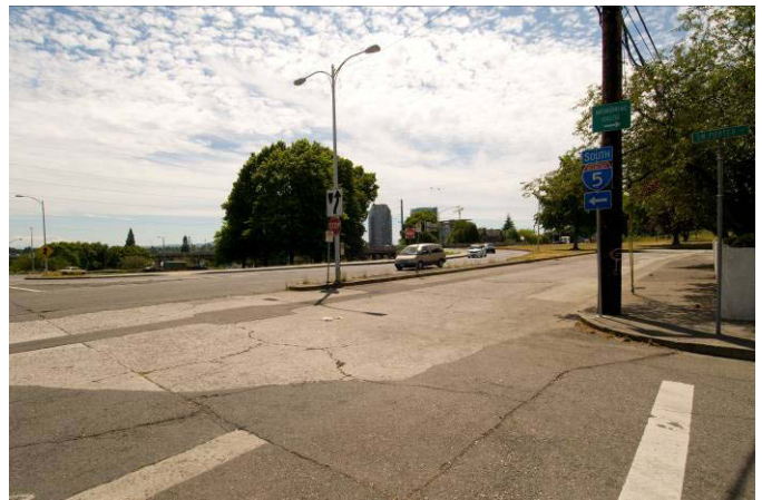
SW Kelly Avenue/SW Porter Street intersection looking southeast. The stop approach for the southbound left turning vehicles can be seen in this photo.
