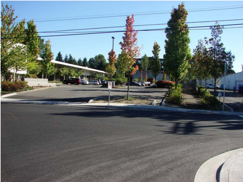
SW Bancroft Street/SW Bond Avenue intersection, looking southbound and the existing dead end. Property would need to be acquired to build Phase II of the South Portal .
