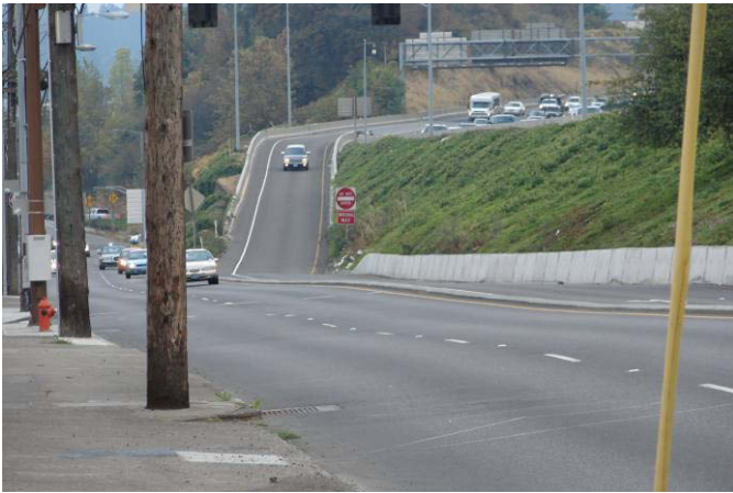
SW Macadam Avenue from near SW Gaines Street looking southbound.
