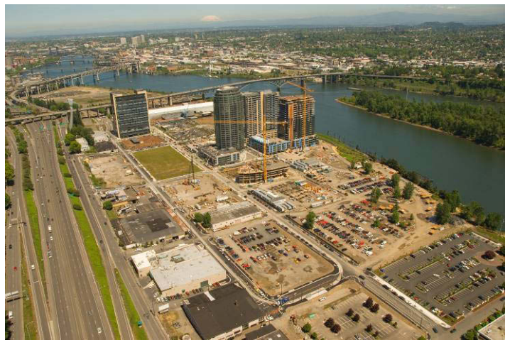
An aerial view of the South Waterfront area including the four intersections that will likely require traffic signals in the future.
