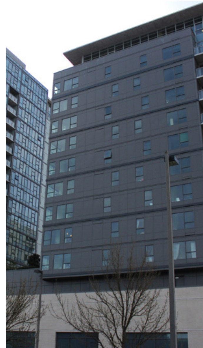
PRIMARY TOWER EXTERIOR - WINDOW WALL
