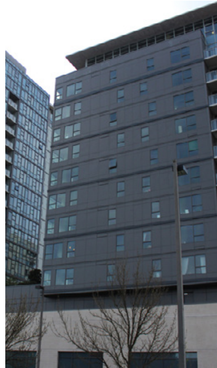
PRIMARY TOWER EXTERIOR - WINDOW WALL
