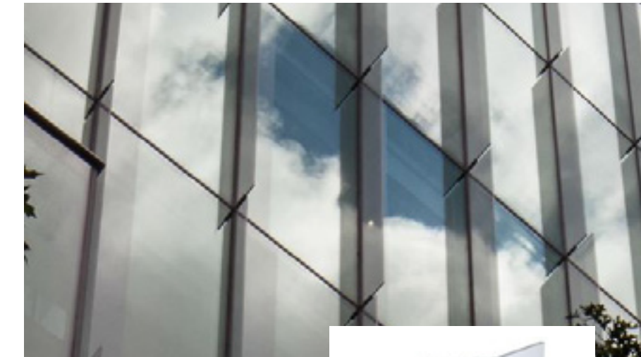
CURTAIN WALL - FOUR-SIDED STRUCTURALLY GLAZED
