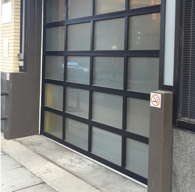
Obscure Panel Sectional Garage Door (Perforated Aluminum not shown)
