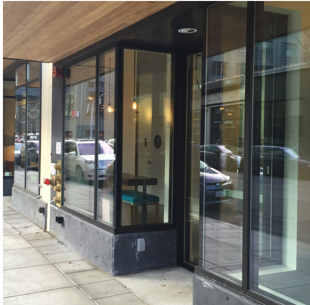
Aluminum Storefront System, Dark Bronze, Front Plane Glazing
