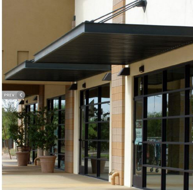
Steel Channel Canopy (Wood Ceiling not shown)
