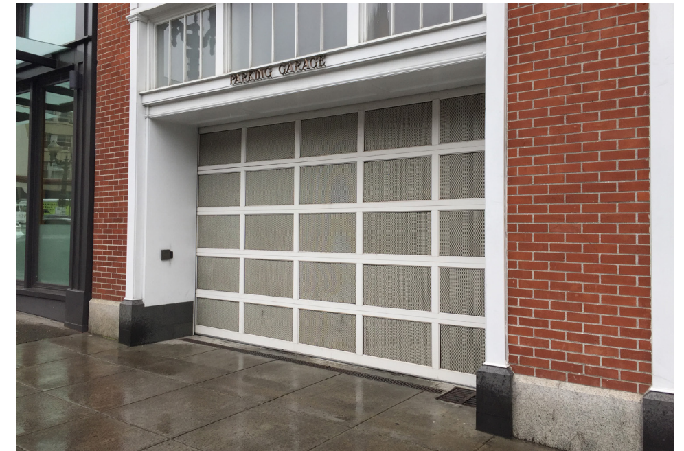
Sectional Garage Door w/ Perforated Panels Panels: 40% Open, 1/8" Dia. Holes, 3/16" Spacing Staggered Telegram Building, Rasmussen/Grace, 1922 - National Register of Historic Places
