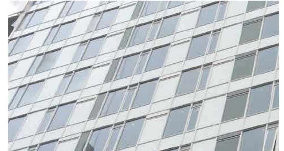
WINDOW WALL 01 - LIGHT GREY METALLIC METAL PANEL
