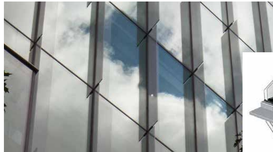
CURTAIN WALL - FOUR-SIDED STRUCTURALLY GLAZED
