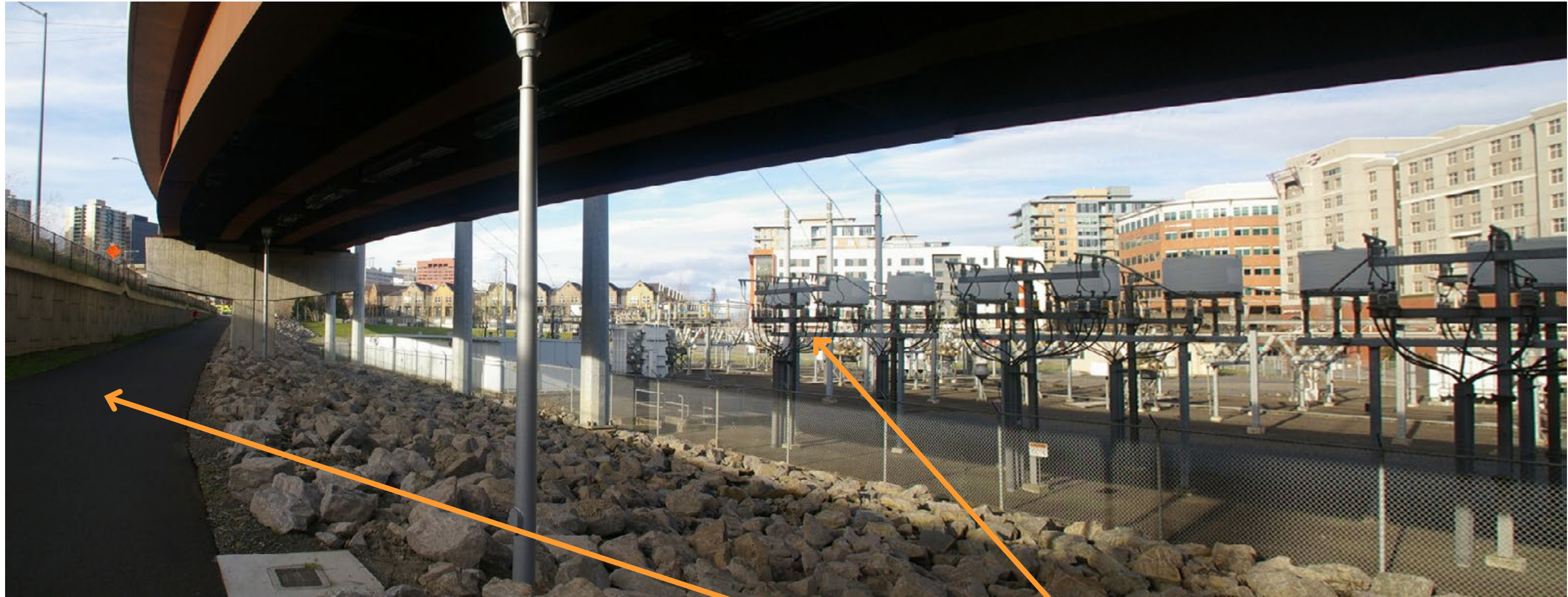
VIEW FROM MOODY AVE LOOKING NORTH FROM WEST PORTION OF BIKE BATH
