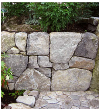
Basalt Retaining Walls
