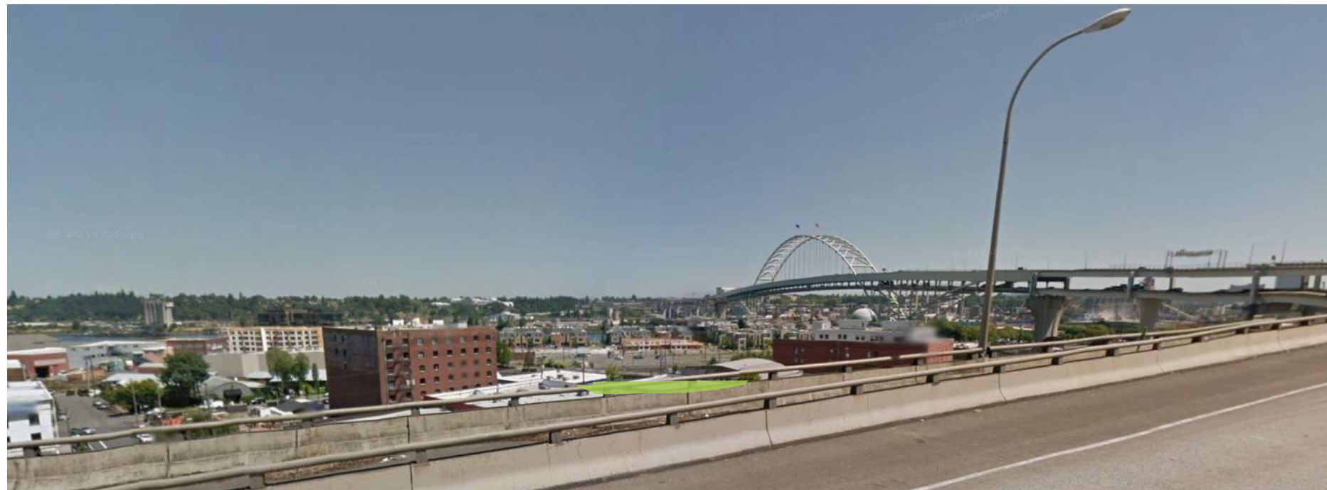
VIEW FROM EXIT RAMP
