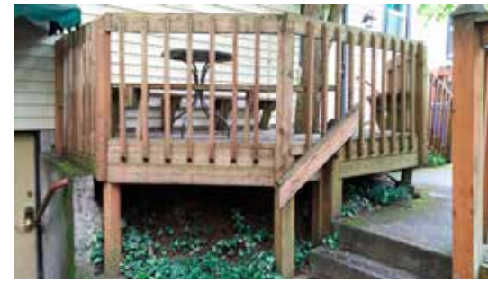
EXISTING DECK IMAGE 1
