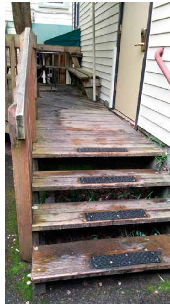
EXISTING DECK IMAGE 3
