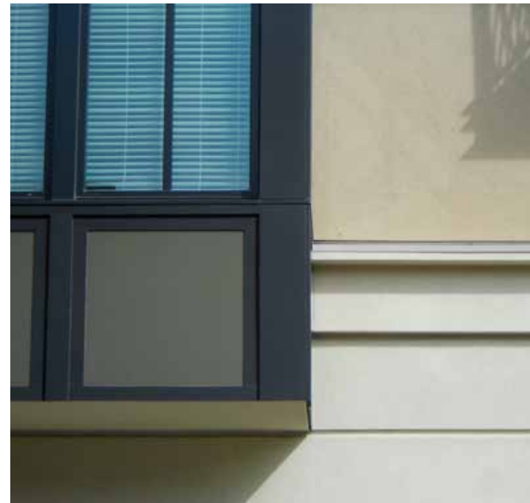
fibercement trim & smooth finish panel at window bay
