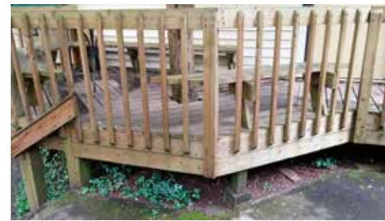
EXISTING DECK IMAGE 2
