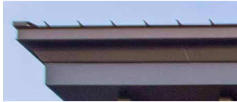
fibercement and metal cornice
