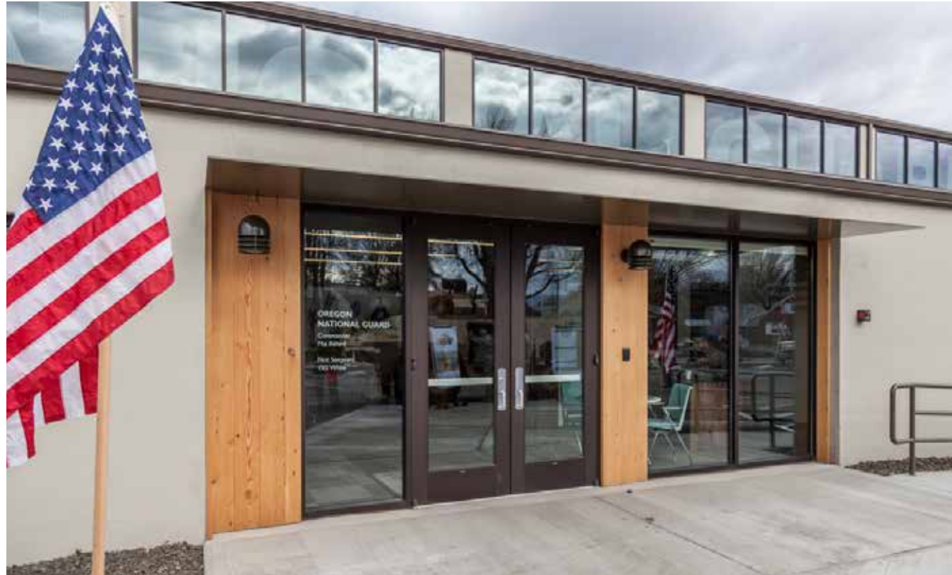
painted steel canopy - shown in historic concrete building
