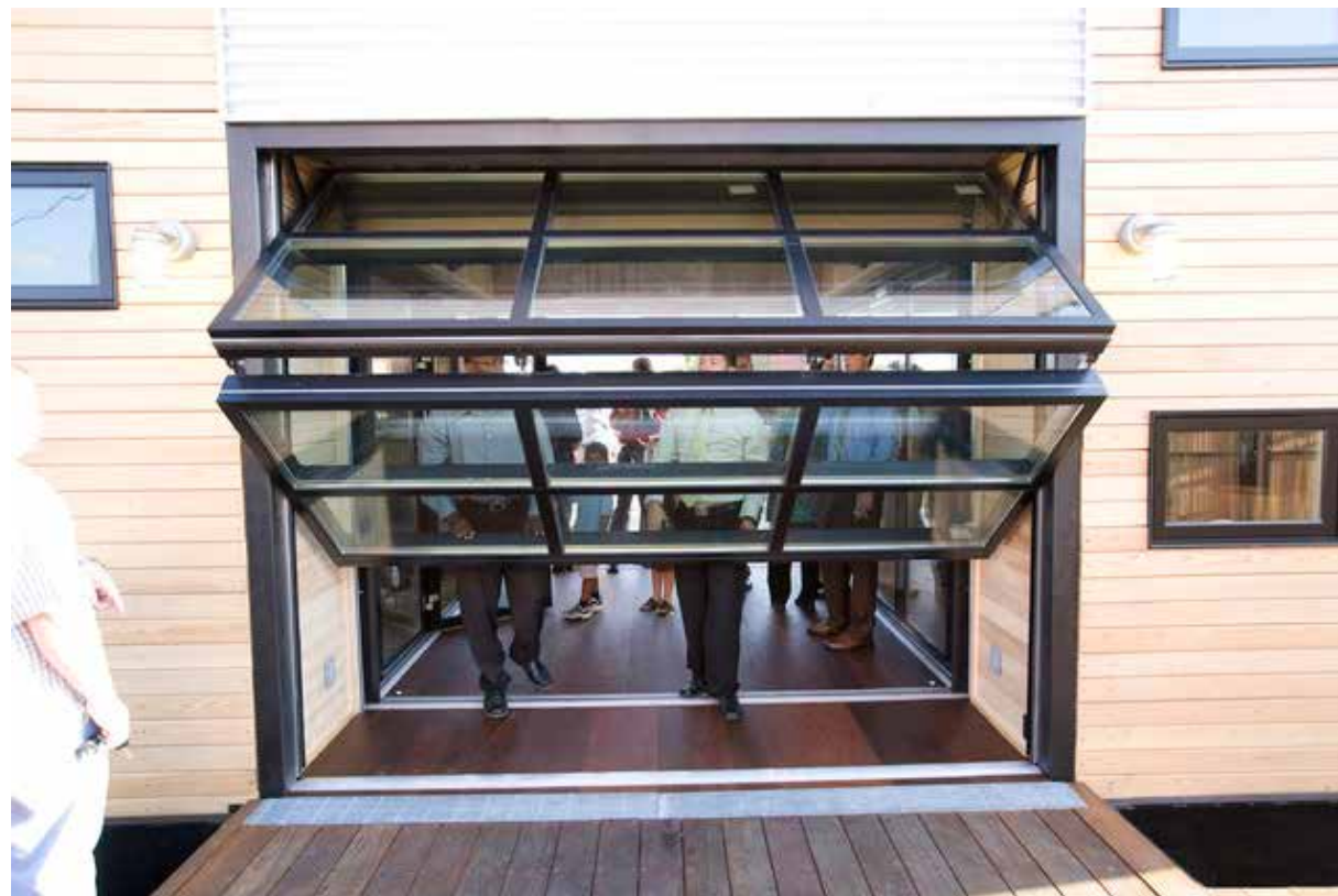
metal garage doors - fold up mechanism
