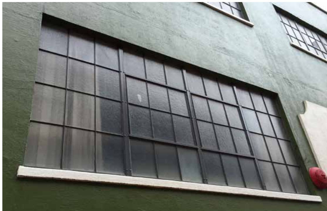
existing steel window
