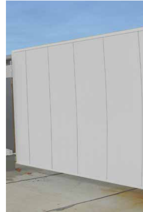
vertical seam metal panel mech screen
