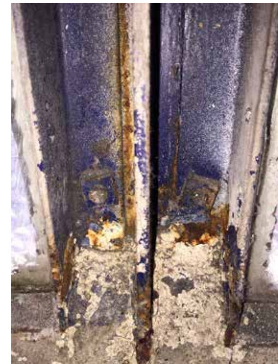
images of existing second floor windows
