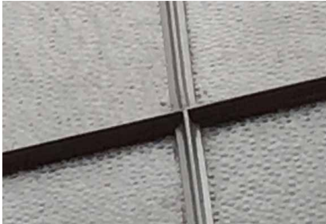
existing steel window mullion
