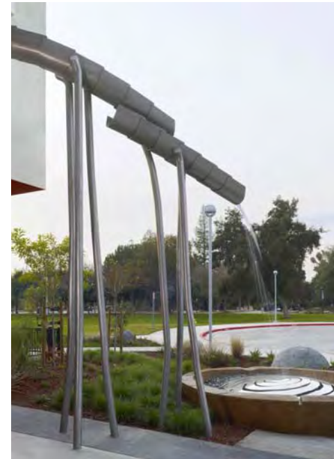
Downspouts cascading water over clear glass cullet encased in steel mesh baskets.
