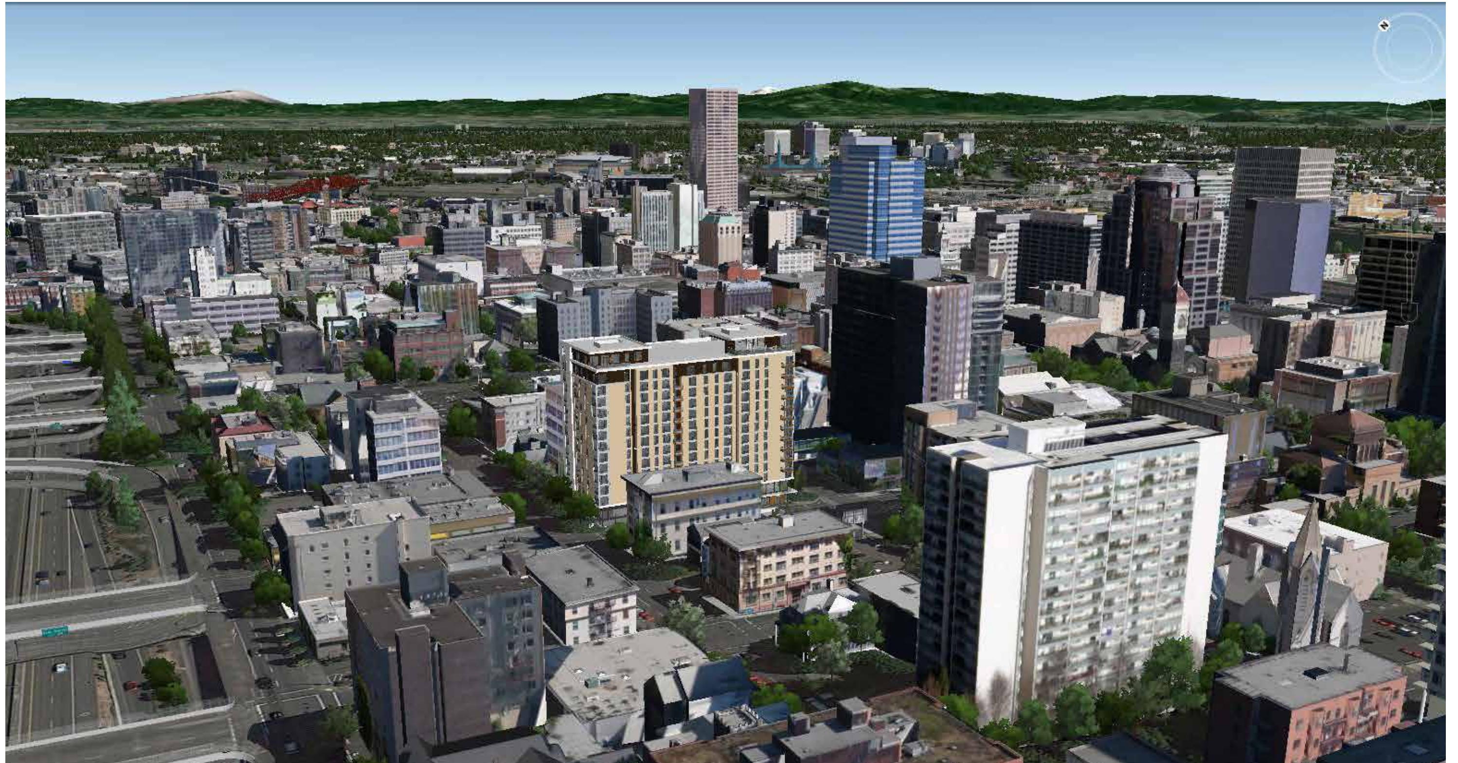
View Northeast of building in City of Portland context
