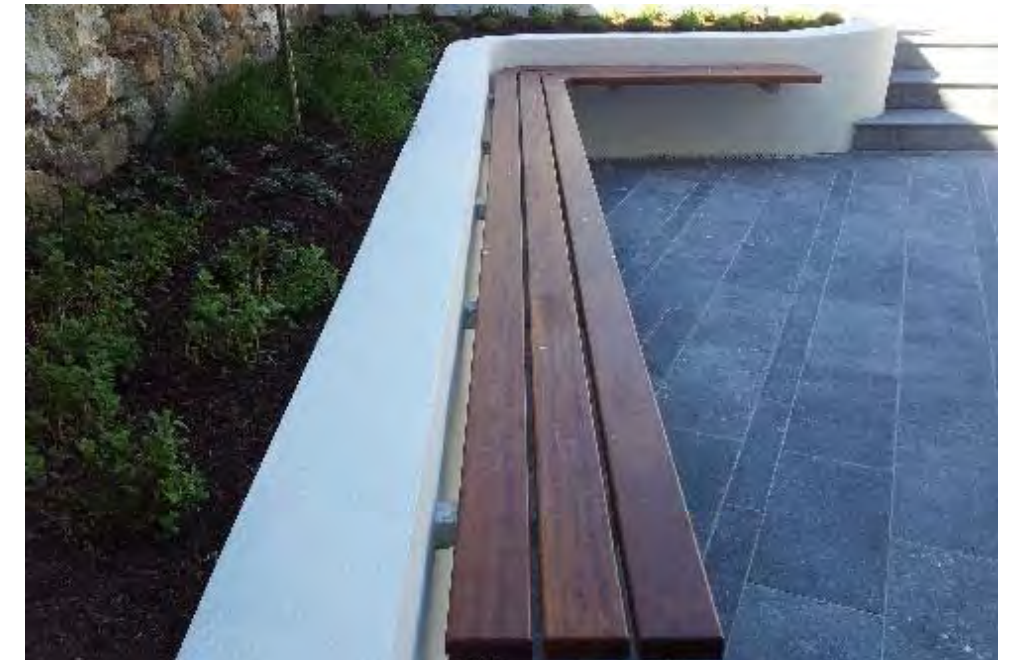
Wood bench mounted to planter wall edge
