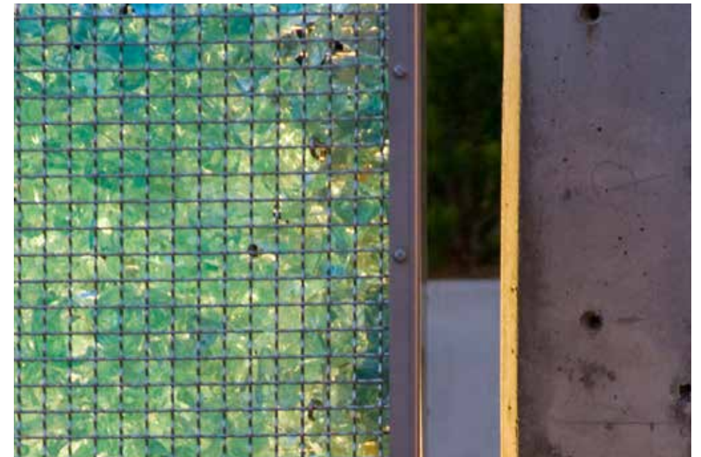
Downspouts cascading water over clear glass cullet encased in steel mesh baskets.
