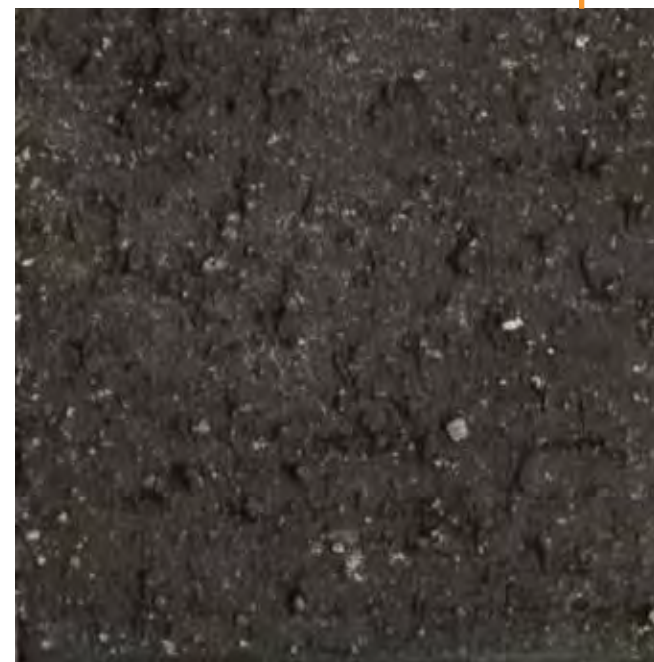
Brick at Ground Level
