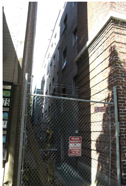
11th looking west at north Property Line / Adjacent Building
