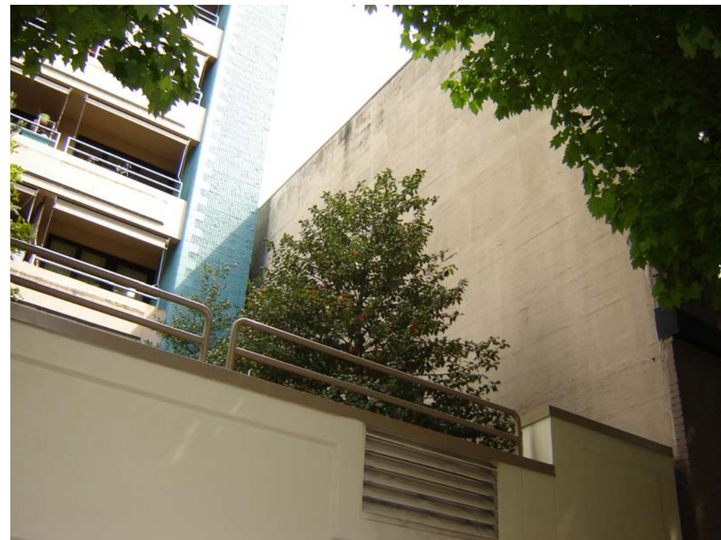
12th looking east at north Property line / Adjacent Building
