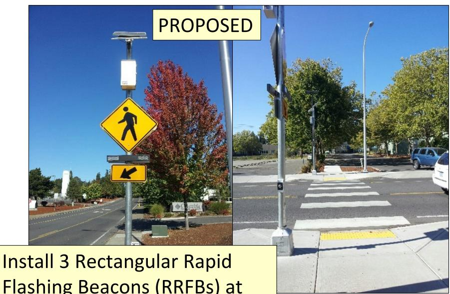
Flashing Beacons (RRFBs) at pedestrian crossings near SE 119<sup>th</sup>, SE 141<sup>st</sup>, and SE 156<sup>th</sup>.
