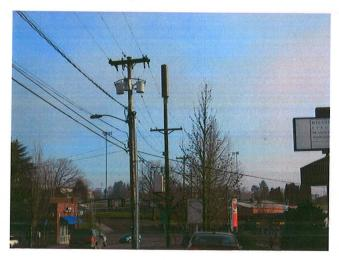
This is an example of a 'micro-cell' located in the SW Sunset Drive right of way near SW Capitol Highway. Please note the wireless facility is behind, and to the right of, the utility pole with three transformers mounted below the top cross arm. This facility provides voice and data telecom services to customers of a major telecommunications provider.
