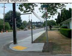
**AFTER**: 6-foot-wide, curb-tight sidewalk with curb ramps. Meets minimum ADA clearance standards at utility poles.
