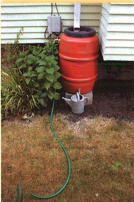
Cisterns that are 6 feet in height or less are allowed in building setbacks. However, cisterns of any size may encroach 20 percent of the depth of the setback.
