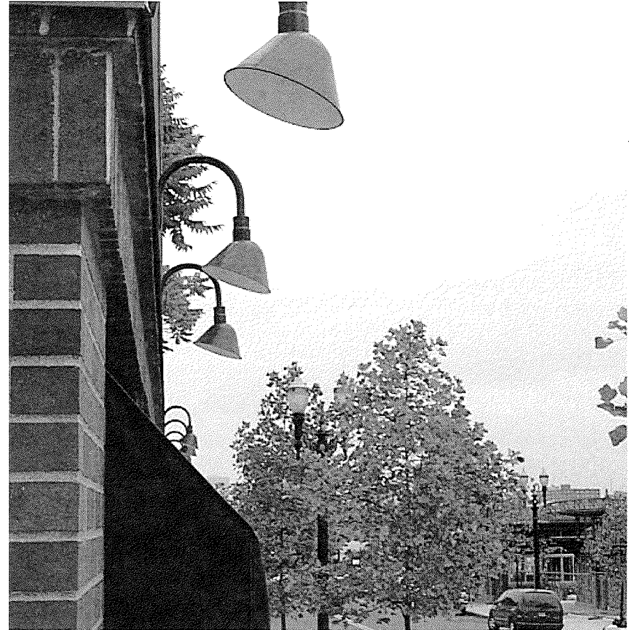
These simple, directional lighting fixtures are attached to a mixed-use development in the RiverPlace community. The fixture's hood helps to shield the light from spreading and directs the light to the sidewalk.
