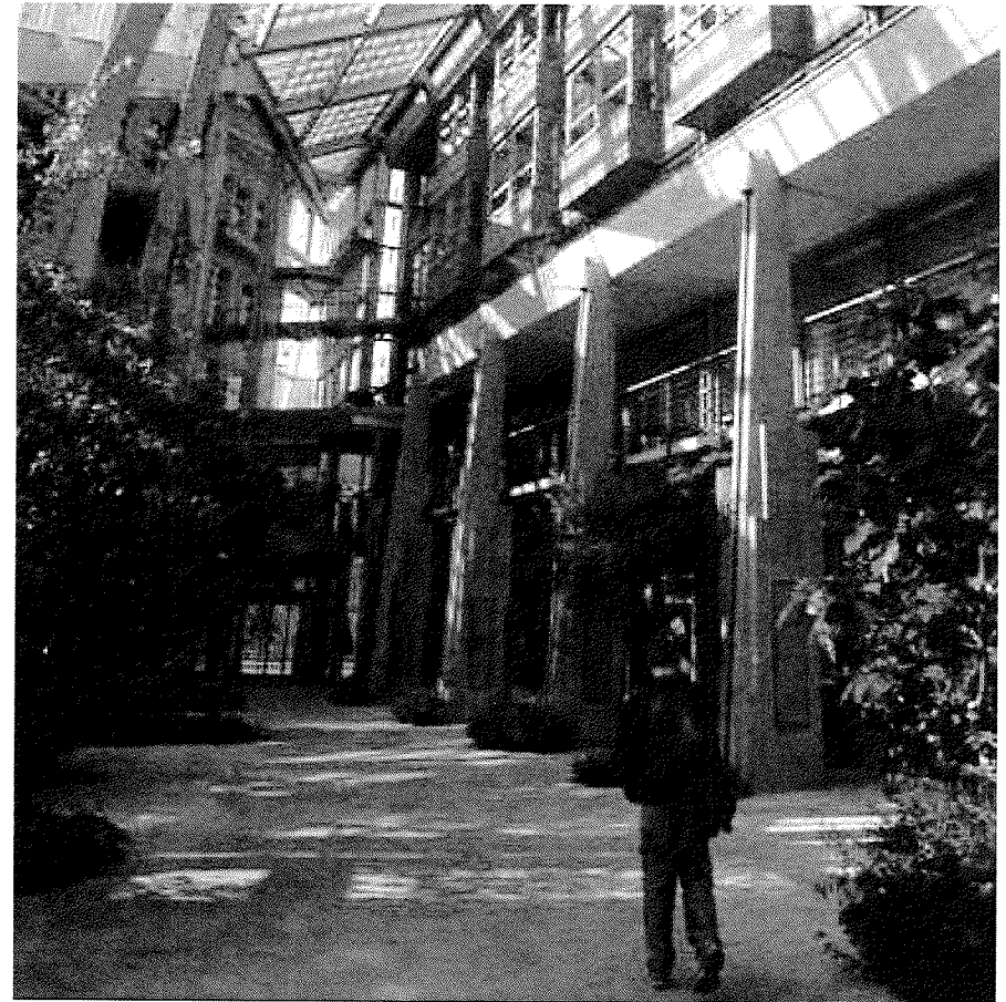
This is an interior view of the sunspace at the Prisma Building in Nuremberg, Germany. This multifunctional space provides a solar heated gathering space for the various tenants of the mixed-use building. It implements passive cooling strategies through plantings and by using water collected outside the building and bringing it inside. These features also strengthen the connections between the exterior and interior environments.
