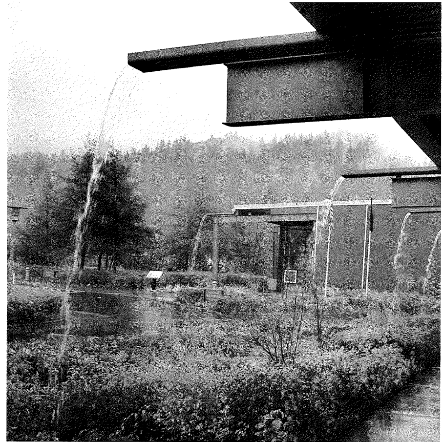
These scuppers at the Water Pollution Control Laboratory have been developed to cascade water from the building's roof into the wetland garden at the northern end of the site. This is a rather poetic and celebratory solution to a typical building element that could otherwise function unnoticed.
