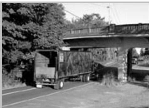
Bertha Blvd. underpass at Capitol Hwy.
