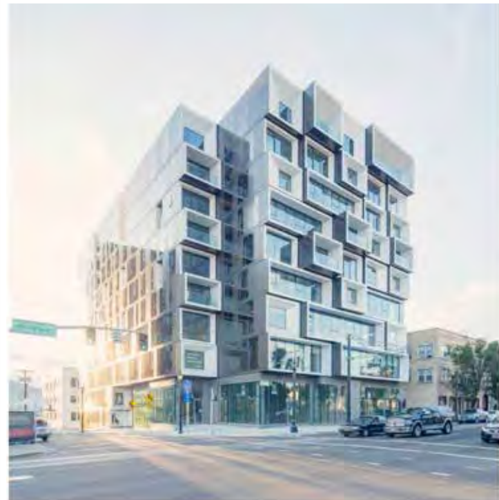
Slate, 10 Floors, 140,000sf
