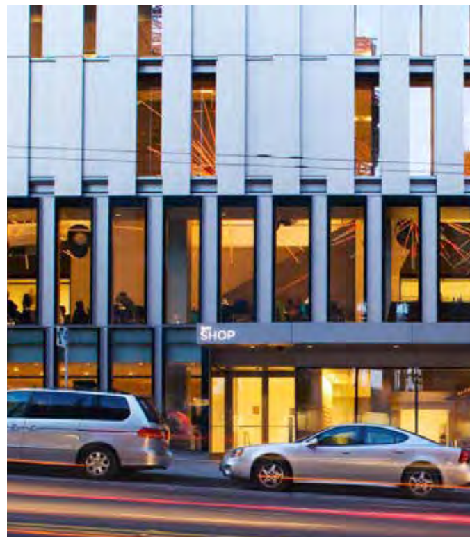
1. Highly Transparent Street Level Facade
