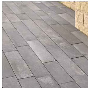
1 CONCRETE PLANK PAVER
