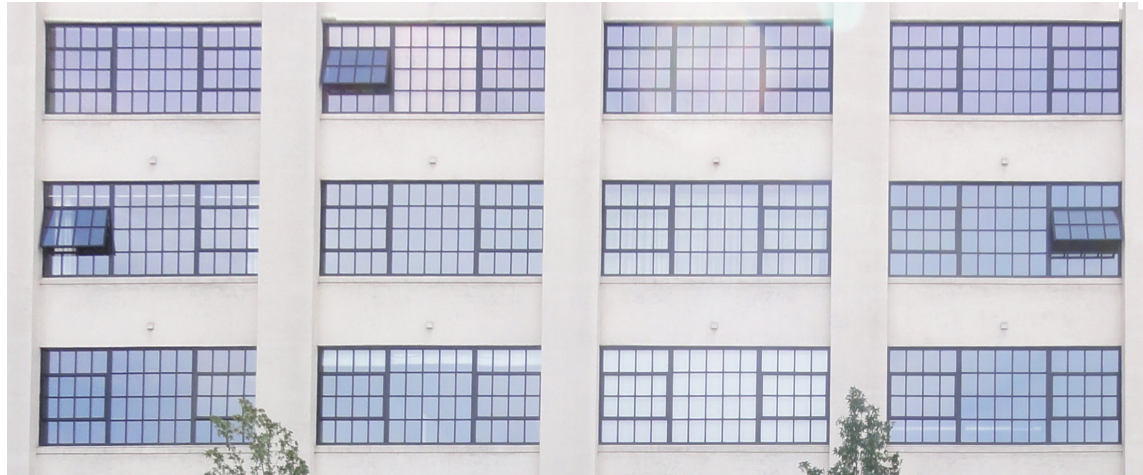
PEARL DISTRICT REINFORCED CONCRETE STRUCTURE
