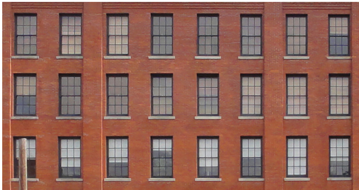
PEARL DISTRICT UNREINFORCED MASONRY STRUCTURE
