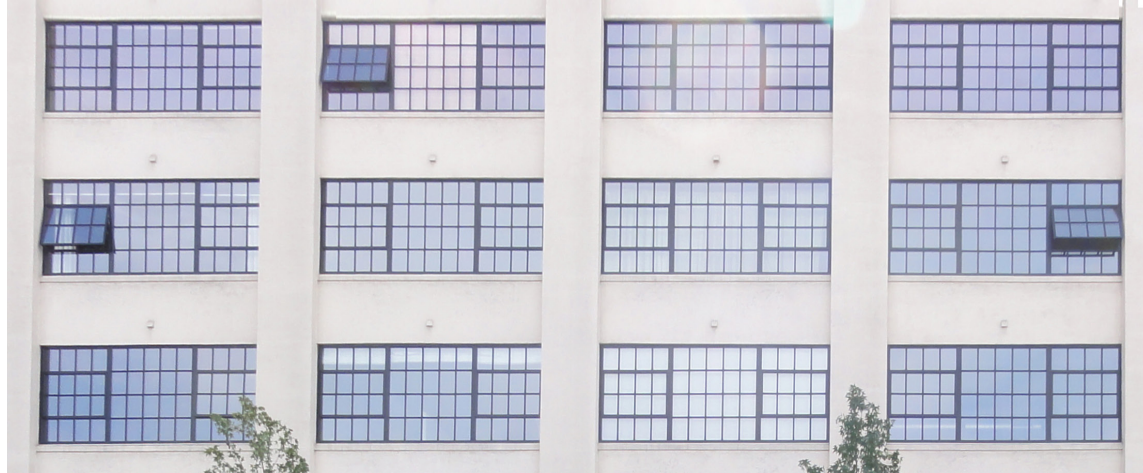
PEARL DISTRICT REINFORCED CONCRETE STRUCTURE
