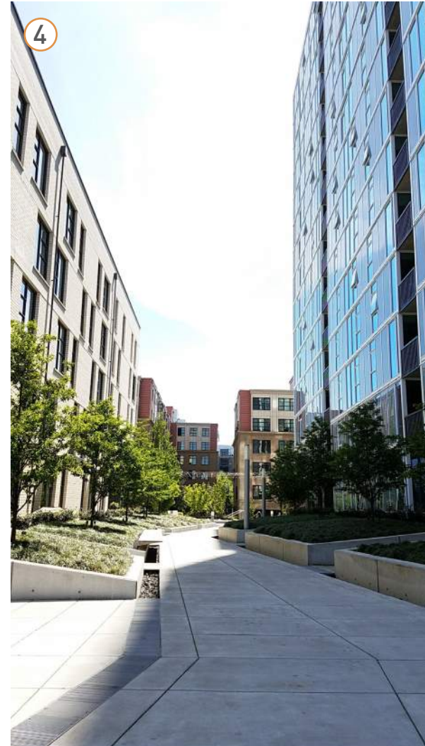
4 BLOCK 17 APARTMENTS | 11th & Overton
