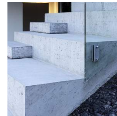
M3. CAST IN PLACE CONCRETE STAIR
