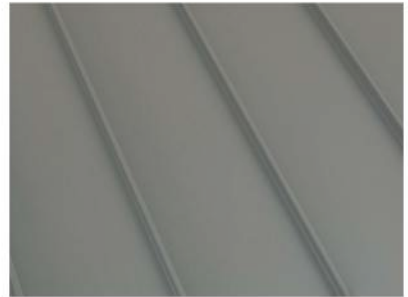
STANDING SEAM METAL ROOFING
