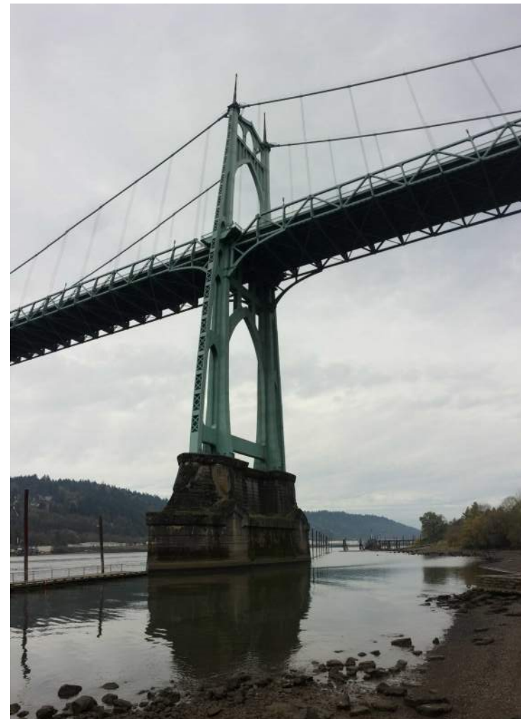
ST JOHNS BRIDGE
