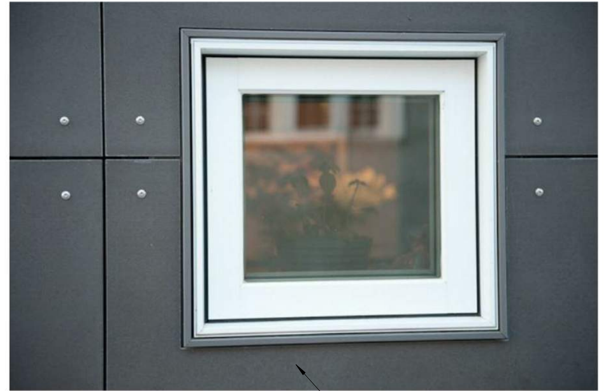
SMOOTH CEMENTITIOUS PANEL; 5/16" THICK; FACTORY COLOR - WHITE; TREATED WITH A UV POLYMERIZING SYSTEM; EXPOSED STAINLESS STEEL PAN HEAD FASTENERS
