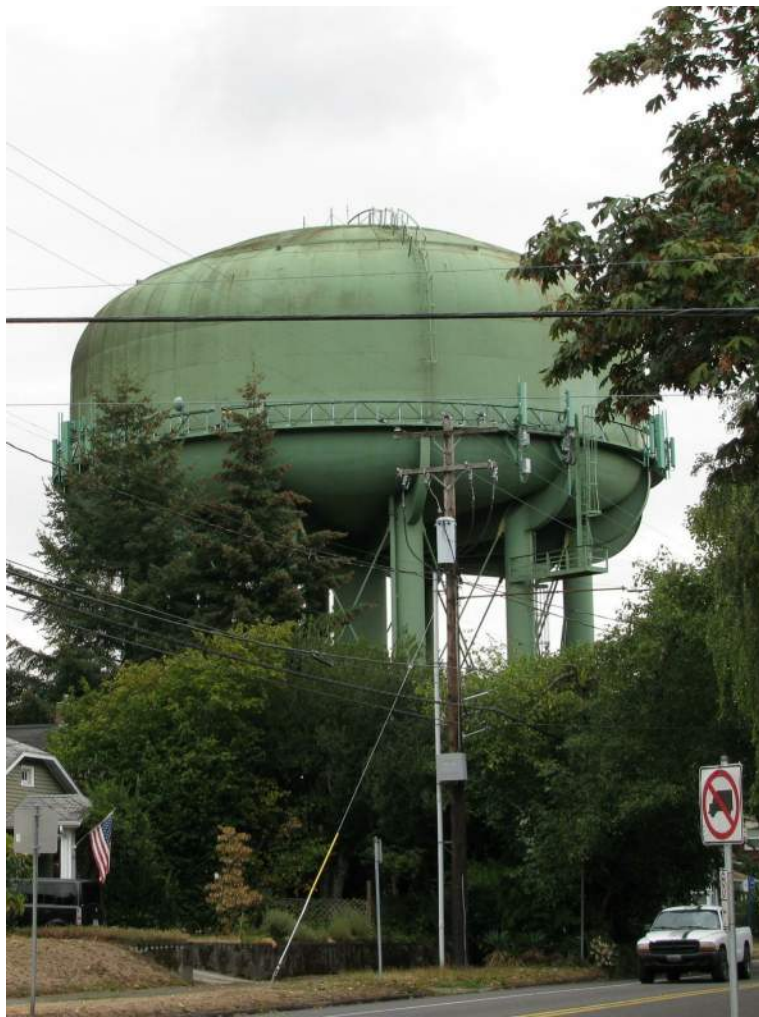
WATER TOWER AT N WILLAMETTE BLVD AND N OSWEGO ST
