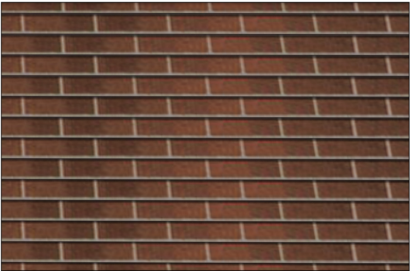
FLASHED RED BRICK norman brick 2.5" x 11.5" xvarying depth running bond
