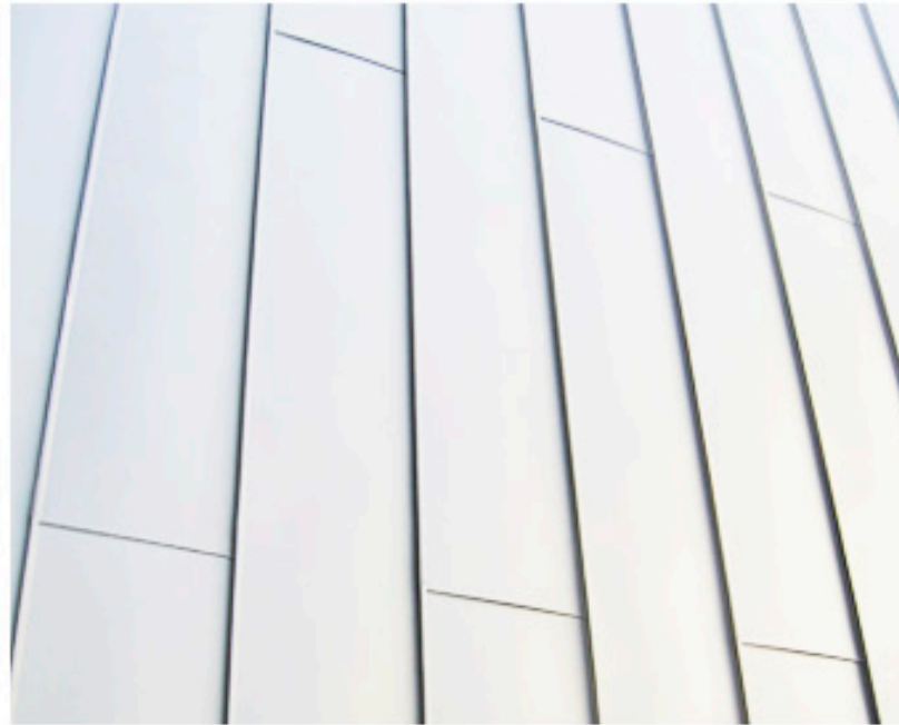
METAL - COATED ALUMINUM STANDING SEAM
