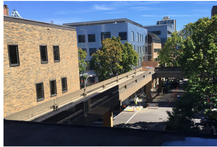
SW BROADWAY PEDESTRIAN BRIDGE FACING EAST
