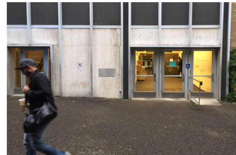
NEUBERGER HALL SOUTH BUILDING ENTRY
