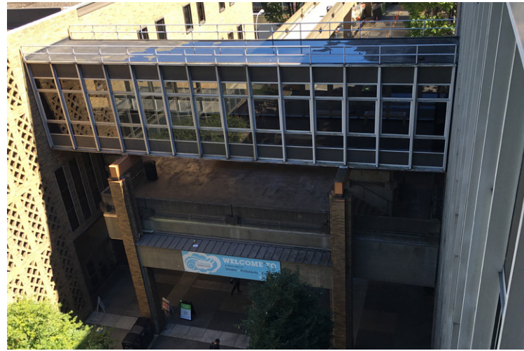
SW HARRISON ST PEDESTRIAN BRIDGES FACING EAST
