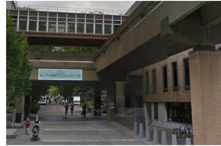
SW HARRISON ST PEDESTRIAN BRIDGES FACING WEST
