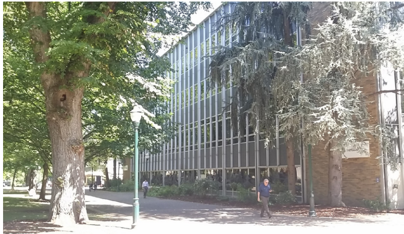
3 NE from Park Blocks
