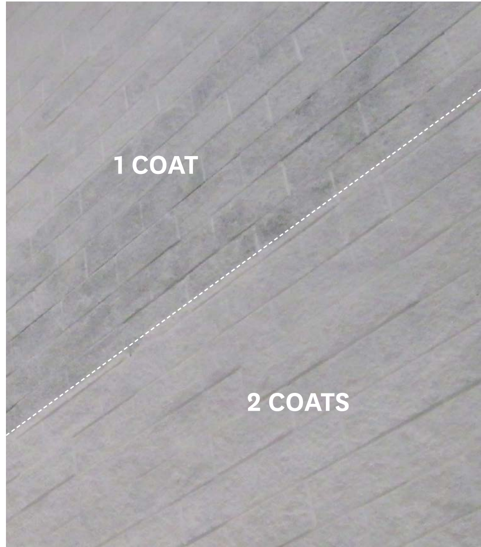
FIGURE B: LIME WASH PROCESS
