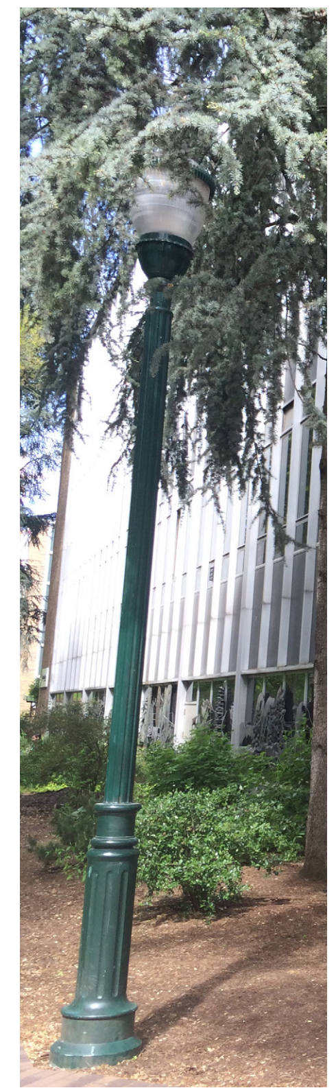
Existing Light Poles to be Reused
