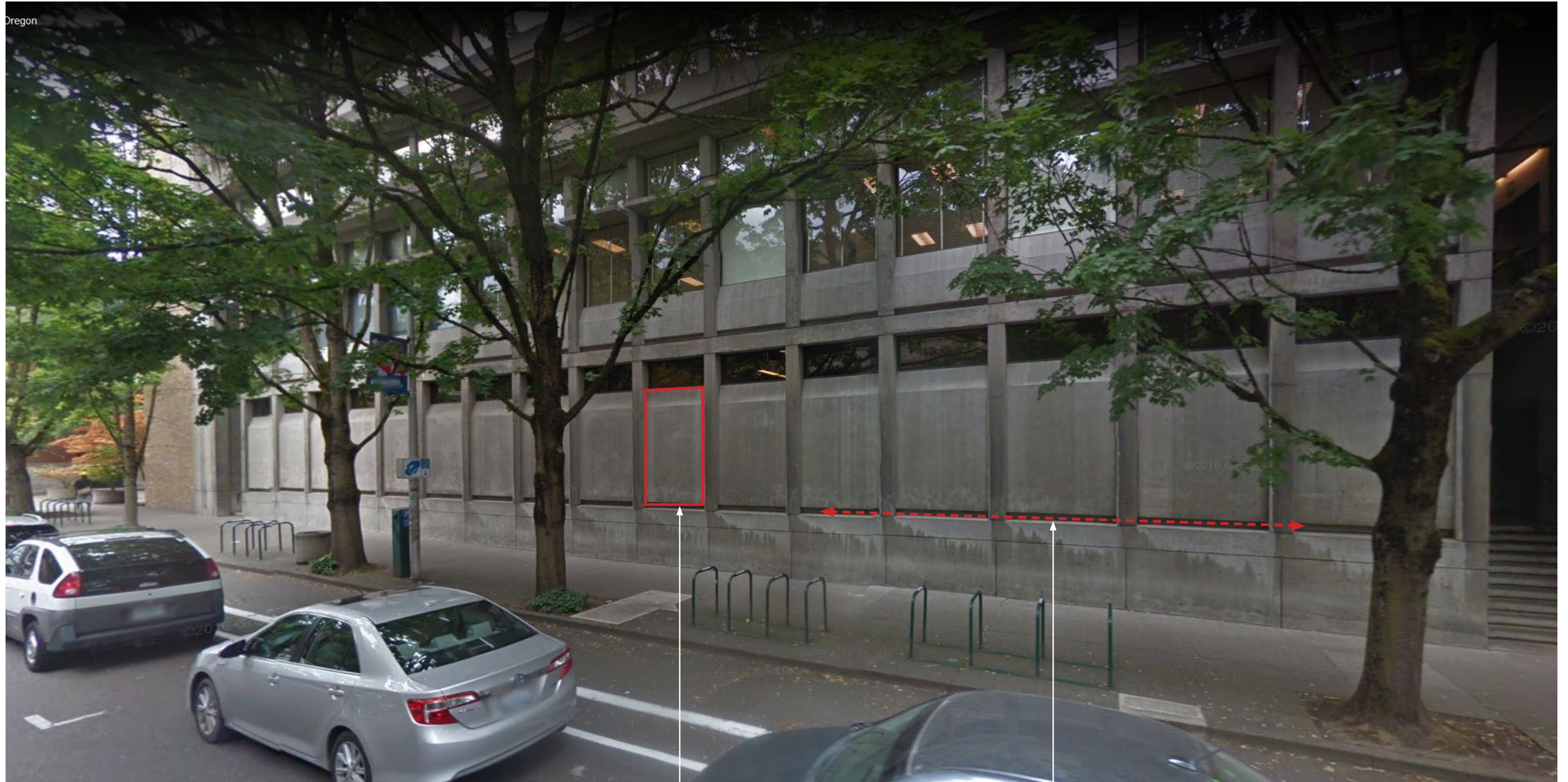
EXISTING EAST FACADE | SW BROADWAY
