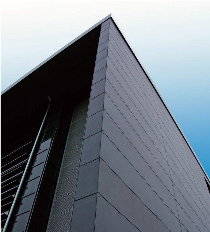
GLASS REINFORCED FIBER CEMENT PANEL Integral Color High Density Painted exposed fasteners
