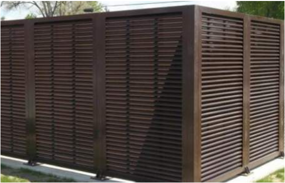
REPRESENTATIVE IMAGE OF LOUVERED SCREEN AT MECHANICAL ROOFTOP
