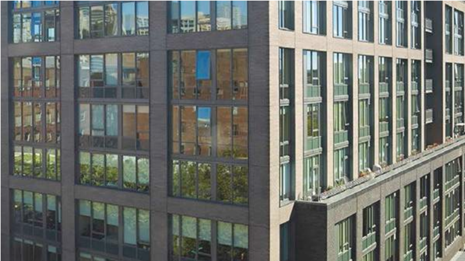
Brick cladding with window wall and brick return (representative image)
