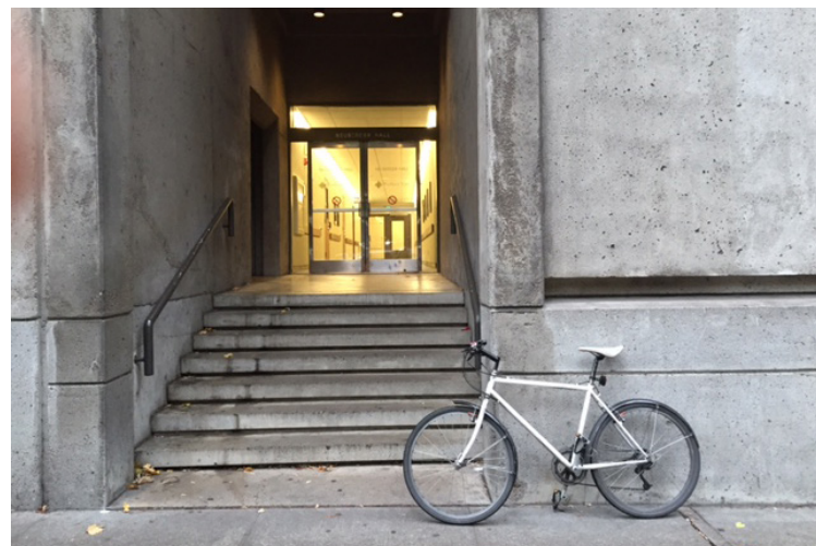
SW BROADWAY EXIT CORRIDOR
