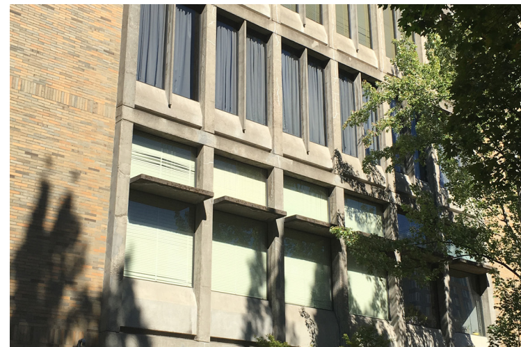
NEUBERGER HALL EAST FACADE GROUND FLOOR
