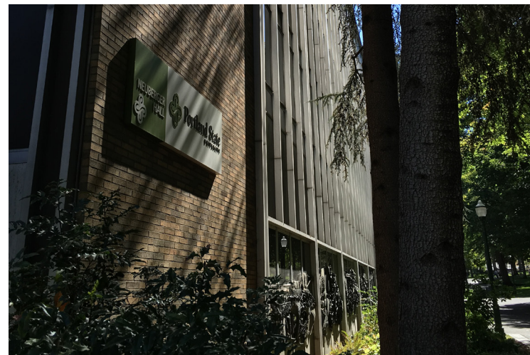
NEUBERGER HALL NORTHWEST FACADE DETAIL
