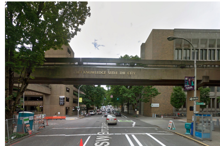
SW BROADWAY FACING SOUTH
