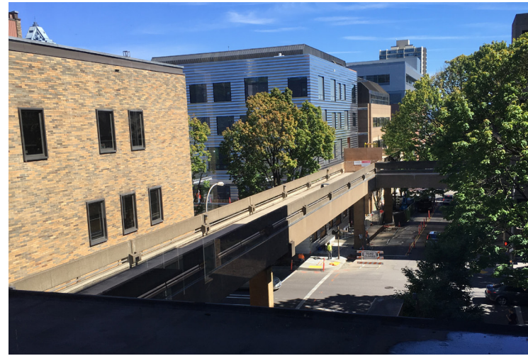
SW BROADWAY PEDESTRIAN BRIDGE FACING EAST
