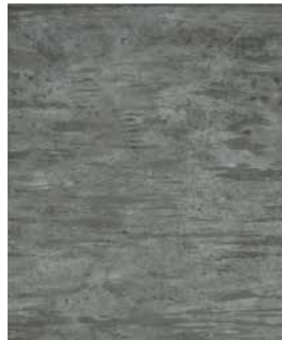
cast in place concrete base
