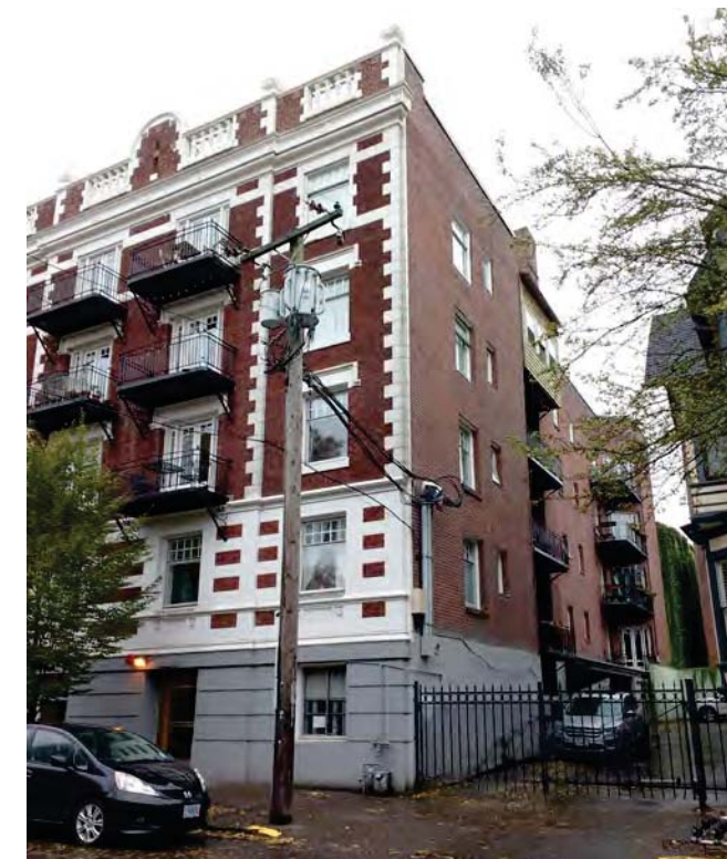
Tudor Arms Apartments, 1915 1811 NW Couch Street, Portland, OR
