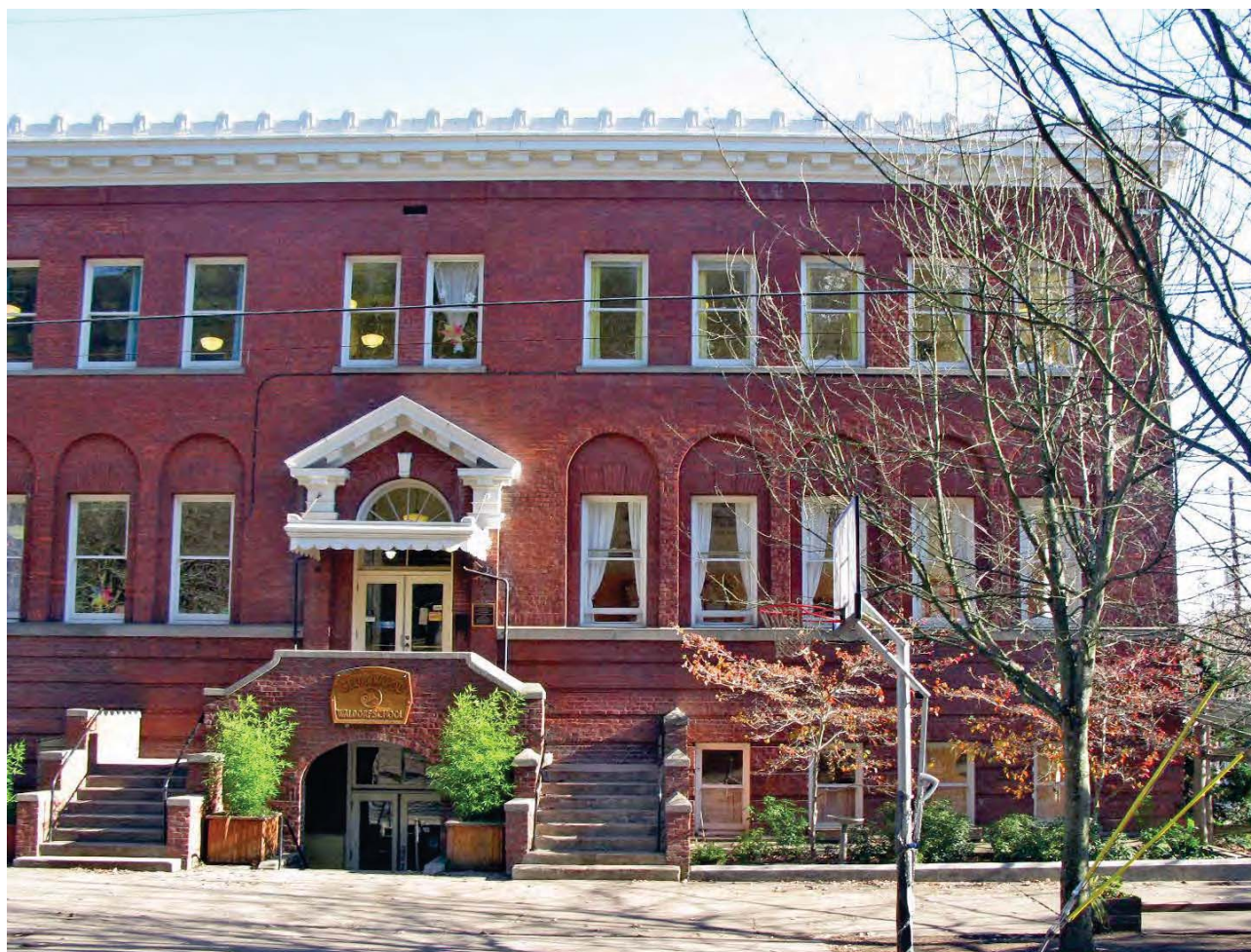
Neighborhood House, 1910 Currently used as Cedarwood Waldorf School 3030 SW 2nd Avenue, Portland, OR
