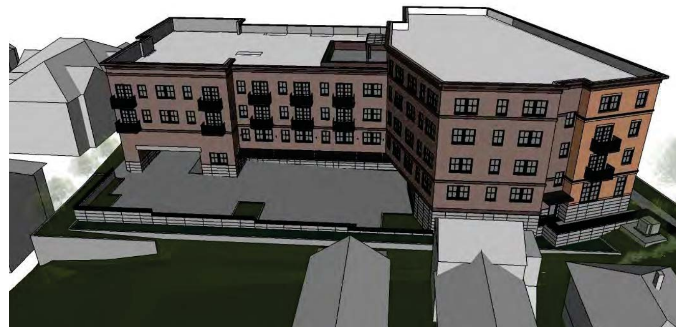
AERIAL OF NORTH SIDE OF BUILDING
